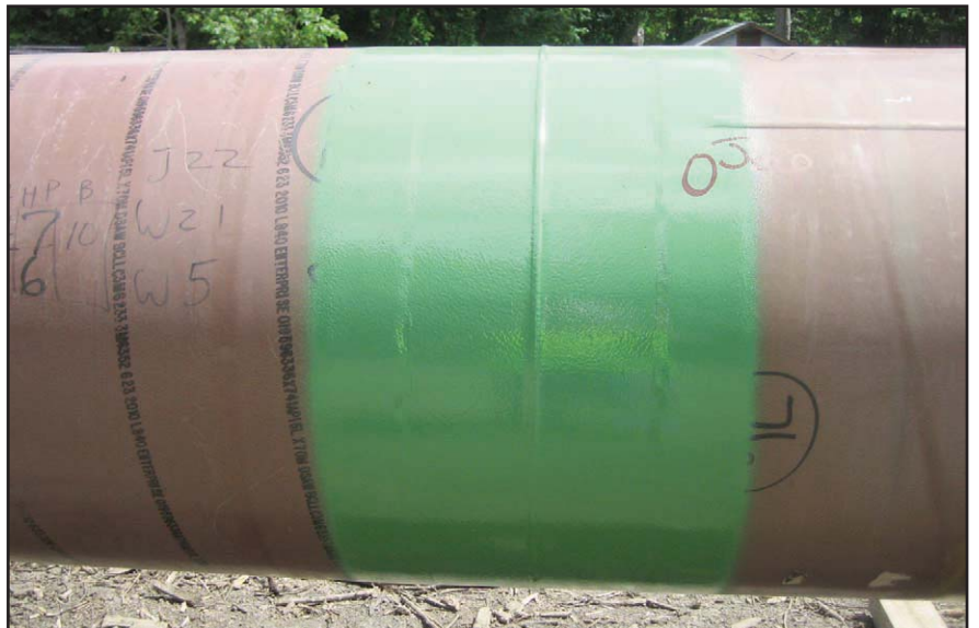
Above: Protal 7200 applied at 24 to 32 mils DFT.
