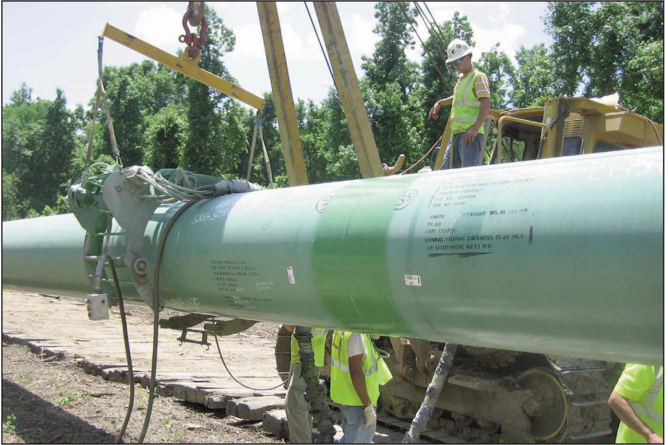
Automatic Spray Ring moving to the next joint.
