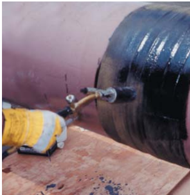
Application of heat on top of Densotherm Tape to seal overlaps.
