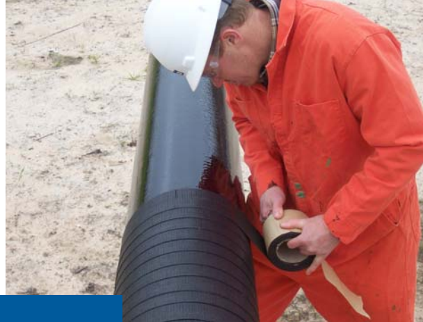
Application of Denso MB-50 Tape.
