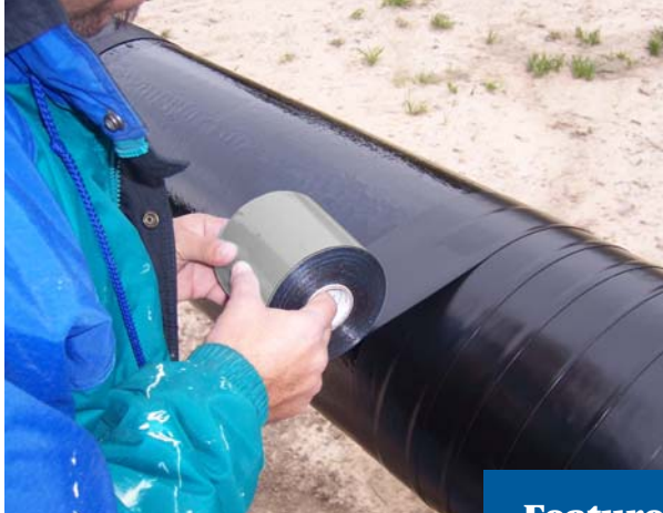
Application of Denso Butyl 35 Tape.
