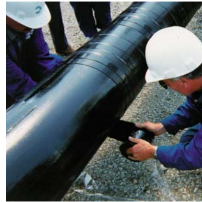
Application of Densopol 60 Tape.
