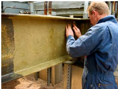
Petrolatum Tape system (Denso Hi-Tack Tape) applied to structural steel.
