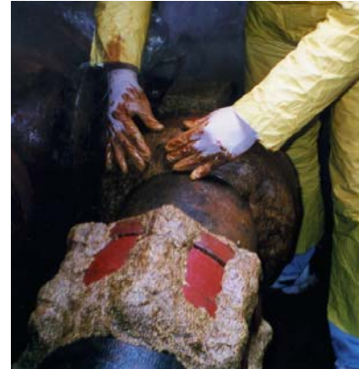
Application of Petrolatum Tape system.
