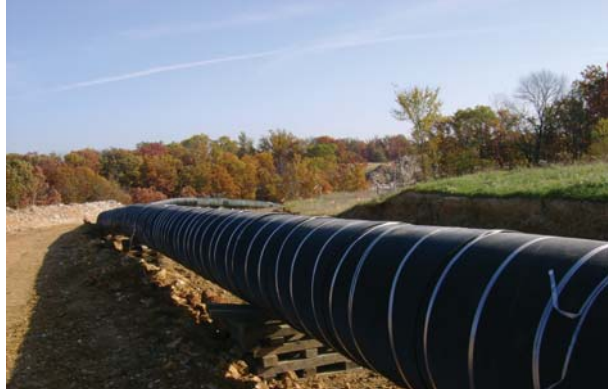
Denso Rock Shield HD is essential where pipelines are constructed through rocky terrain.
