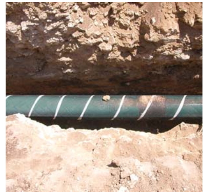
Denso Rock Shield SD in action, protecting the pipe coating.
