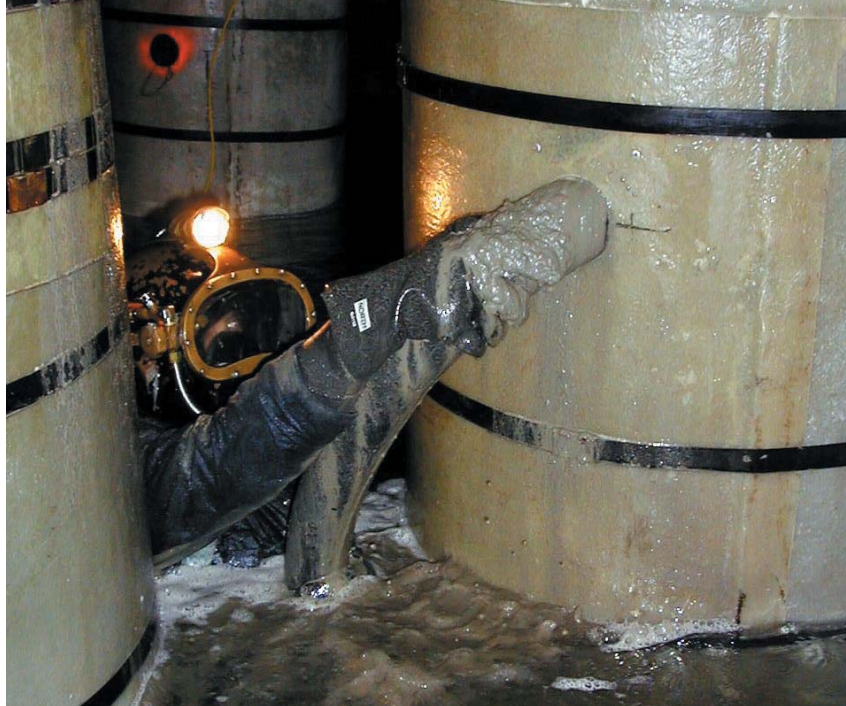
Structurally repaired timber piles with rebar, concrete and translucent SeaShield Fiber-Form fiberglass pile jackets.
