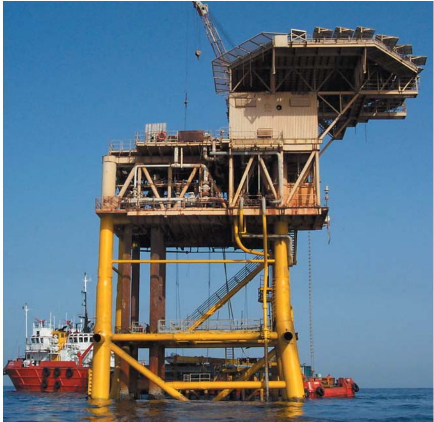
The one-coat glass flake reinforced polyester coating which can be applied by airless spray to achieve a dry film thickness of 30 - 40 mils in a single coat.
