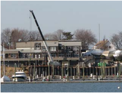
Tern Harbor Marina in Weymouth, MA where the old corroded timber was replaced with new Rigspray coated steel sheet piles.
