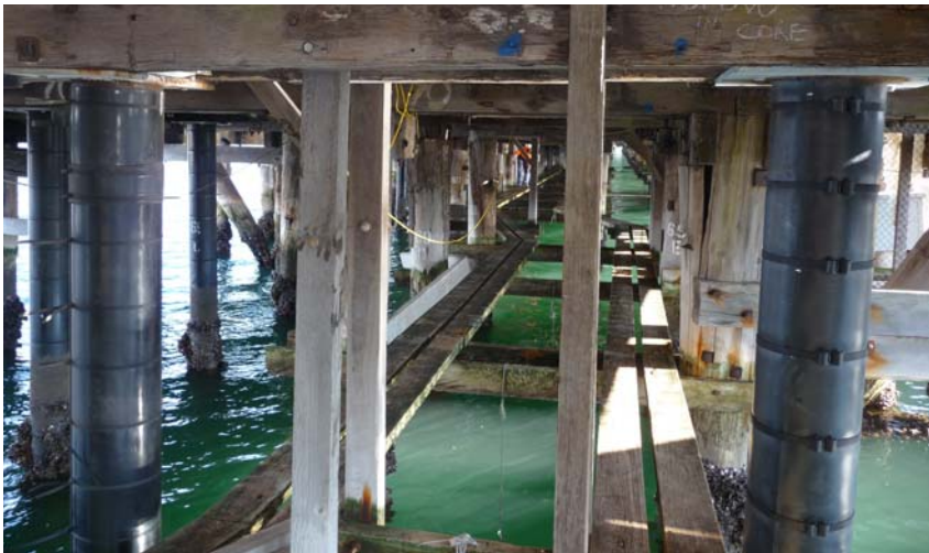
▲ The components of the Series 100 System can be applied under water with minimal surface preparation. ▼
