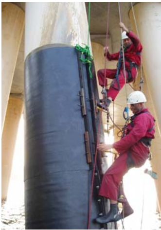
The SeaShield Series 2000FD System features a controlled application tensioning system.
