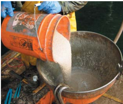
SeaShield 550 Epoxy grout being mixed and poured into pump.
