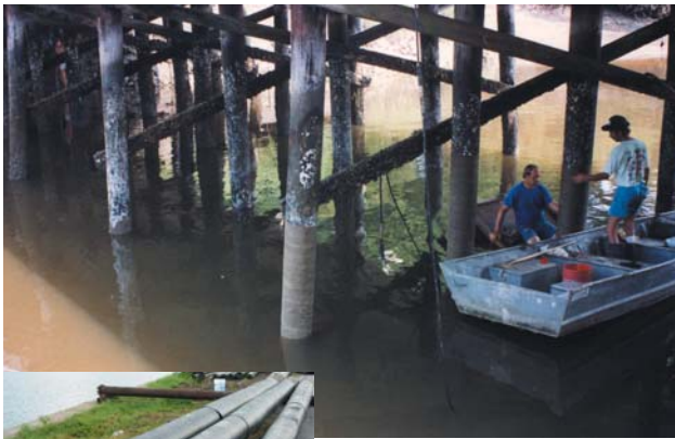
SeaShield Series 90 consists of Denso Marine Piling Tape preventing marine borer destruction and an outcover for mechanical protection of tape.
