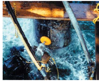
▲ The components of the Series 100 System can be applied under water with minimal surface preparation. ▼
