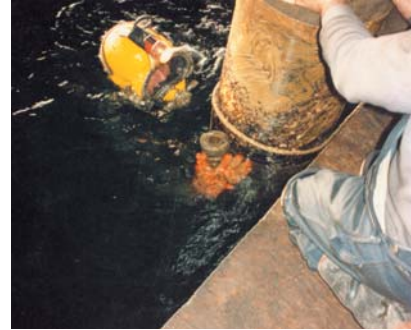
▲ The components of the Series 100 System can be applied under water with minimal surface preparation. ▼
