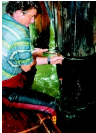
The SeaShield Series 30 System can be applied to both new and existing timber piles. The unique design provides an effective solution for the prevention of marine borer infestation.
