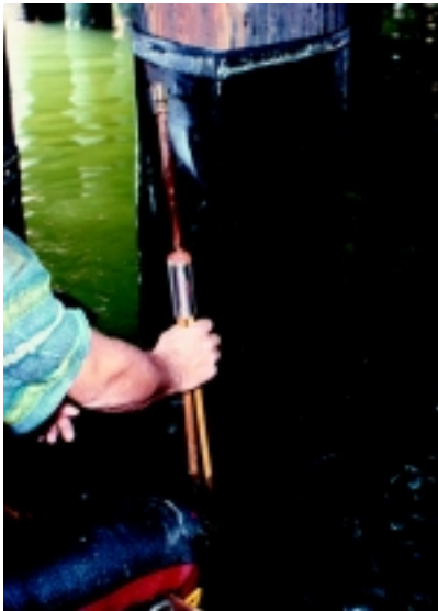
The SeaShield Series 30 System can be applied to both new and existing timber piles. The unique design provides an effective solution for the prevention of marine borer infestation.
