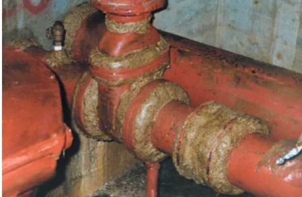
Denso Profiling Mastic on valve and coupling.
