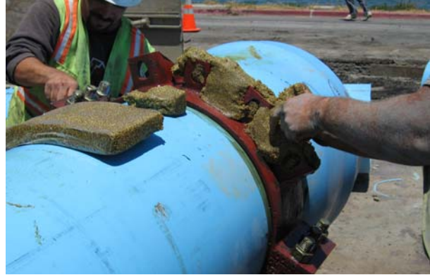
Coupling prepared with Denso Paste and Profiling Mastic prior to Petrolatum Tape.
