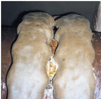
Densyl Mastic Blankets applied to flange pair.
