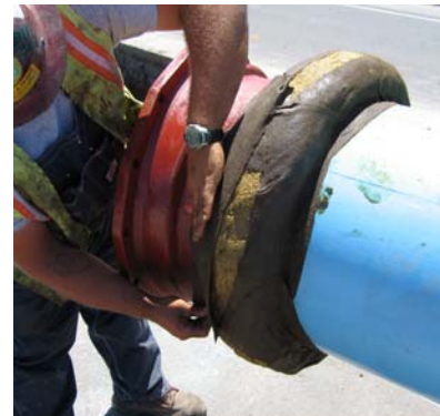
Denso Profiling Mastic and Densyl Tape applied to coupling.
