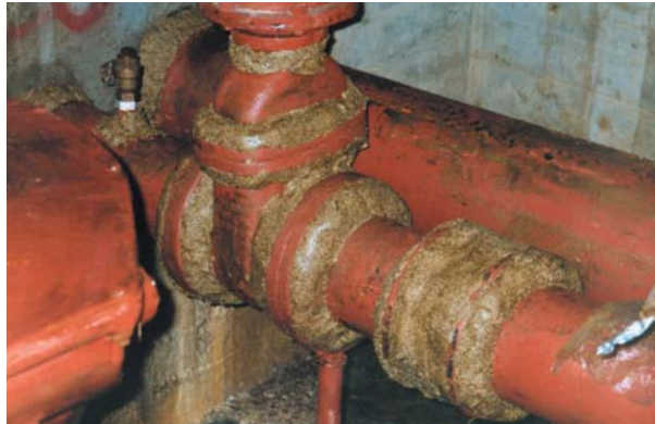
Denso Profiling Mastic on valve and coupling.
