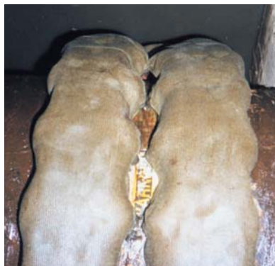
Densyl Mastic Blankets applied to flange pair.
