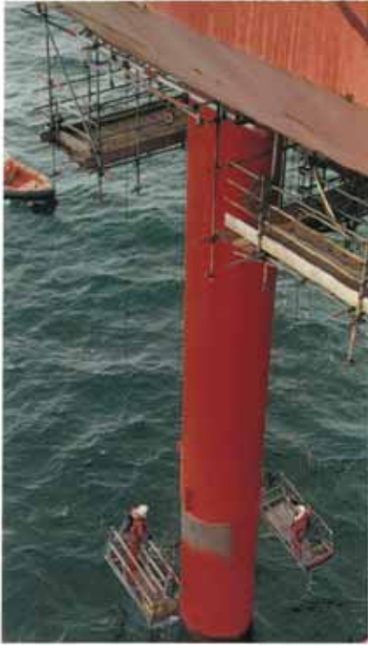
In-situ application of Rigspray.
