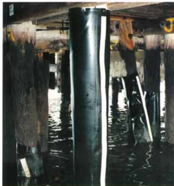
Installation of system in progress.
