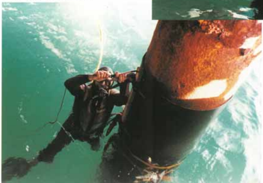
Connection of power supply prior to electrofusion.
