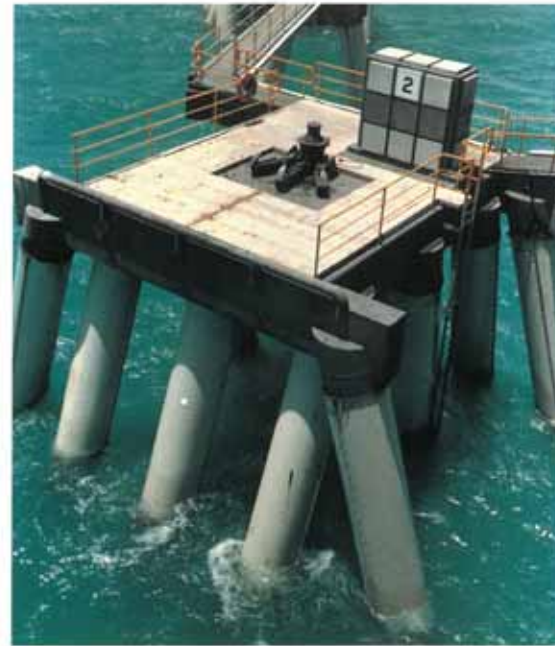
SeaShield 300 System installed on berthing dolphin at Abbot Point.
