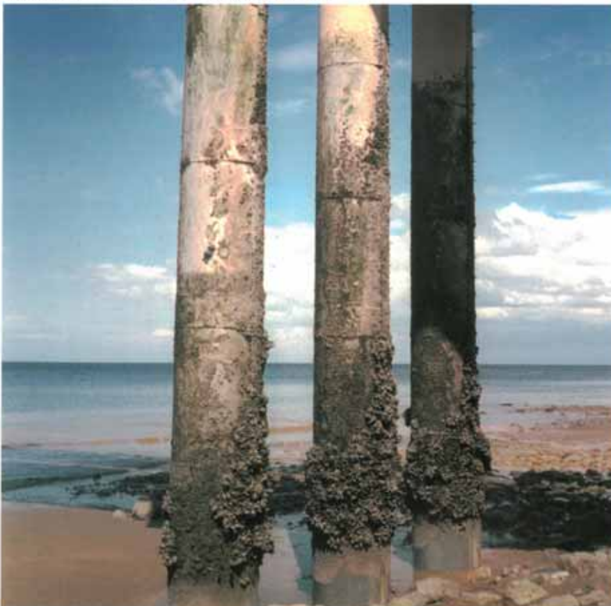
Inspection May 1995 - marine growth on SeaShield jackets after 10 years.
