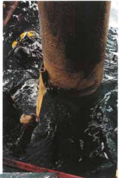
Application of petroleum tape.
