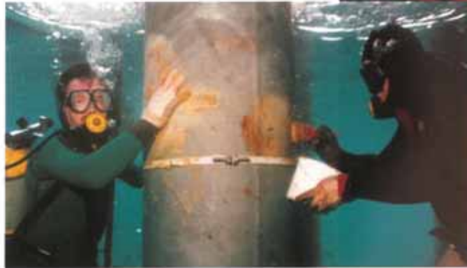
Application of petroleum tape.
