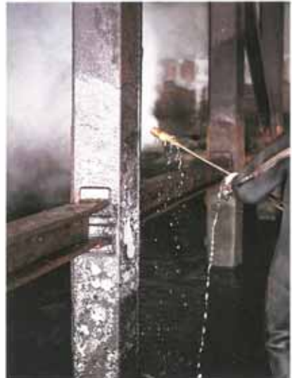
H.P. water jet cleaning using a Neolith SP2 rotating head at 12,000 psi.
