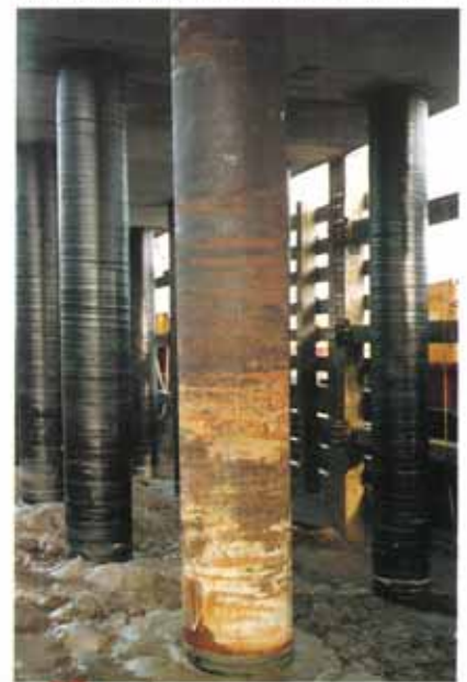
Prepared pile before installation of SeaShield Series 80 System.
