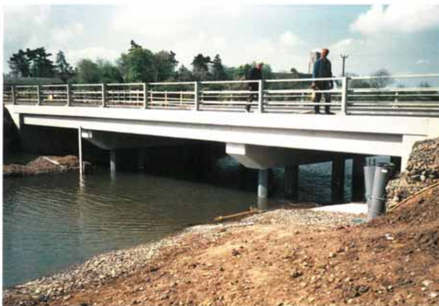
View of bridge during jacket installation.
