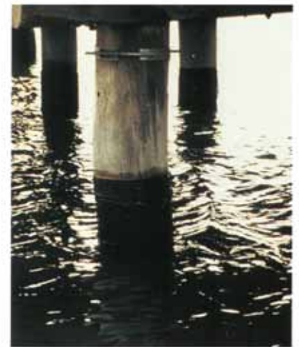
Road bridge no.3438, completed installation of SeaShield Series 60 System with Pilemesh.
