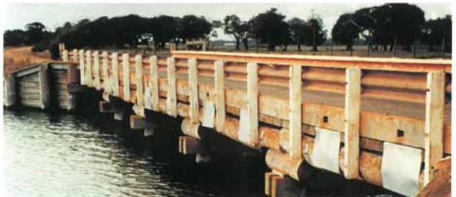
Road bridge no.3447A, twelve 500mm diameter timber pile protected
