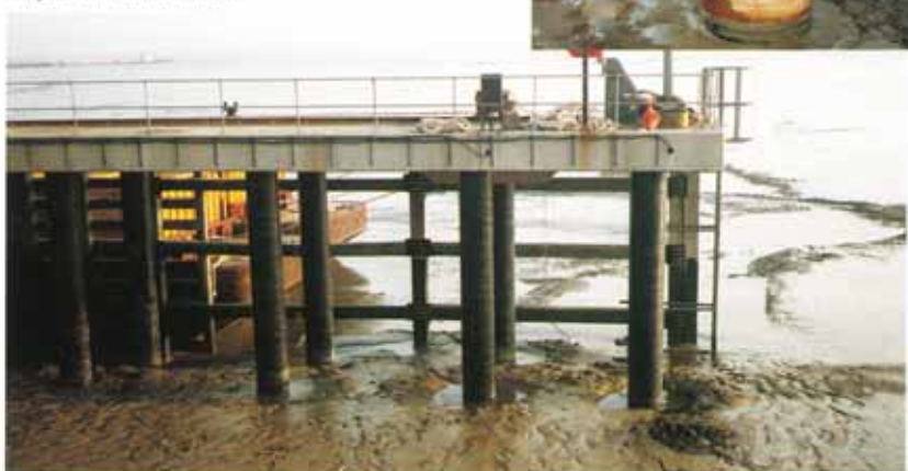
Completed installation at low tide.
