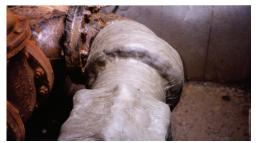
Fully protected coupling and flange with the Denso Petrolatum Tape System.
