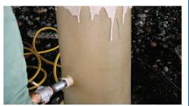
SeaShield  $^{\scriptscriptstyle\rm TM}$  550 Epoxy Grout being pumped into the Fiber-Form jacket.
