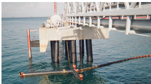
SeaShield™ Series 2000HD System installed on the pilings at the Decal Panama.
