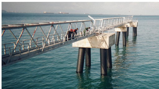
Pumping 550 Epoxy Grout underwater in a Denso Round Fiber Form.
