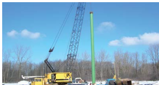
A steel air shaft is welded to a tunnel section prior to the Protal application.
