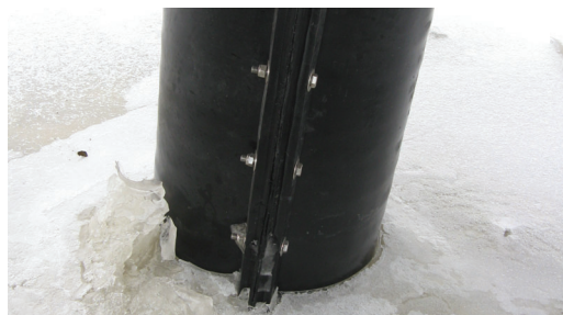
SeaShield™ Series 2000HD protecting a steel pile during winter ice build up.
