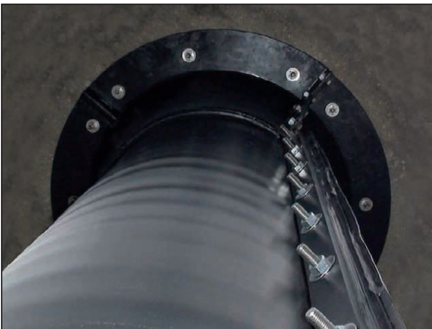
View of the underside of the jetty deck, shows the complete encapsulation and degree of protection given to the pile with the use of this system .
