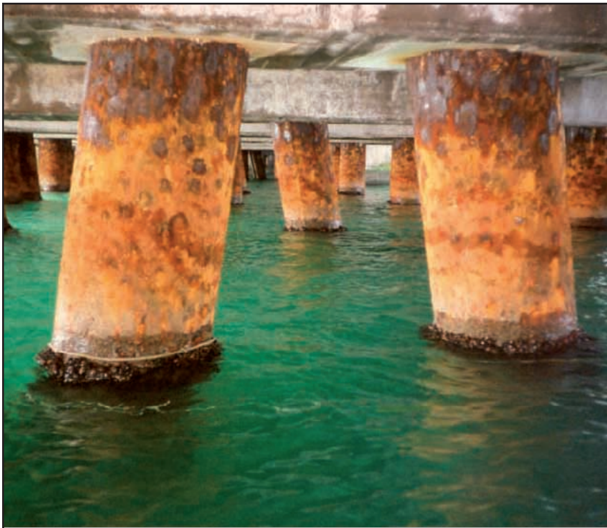
Cleaned piles ready for the application of the Petrolatum Inner Layer.
