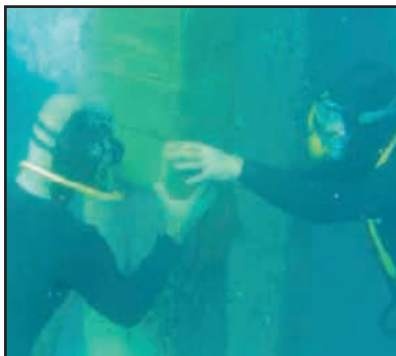
Tape application underwater
