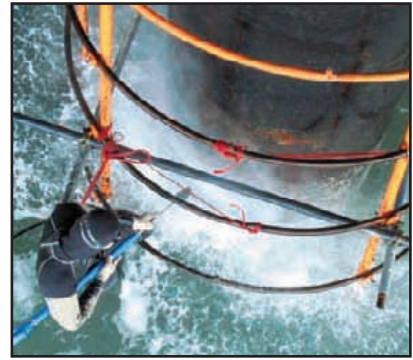
Cleaning using a high pressure water jet
