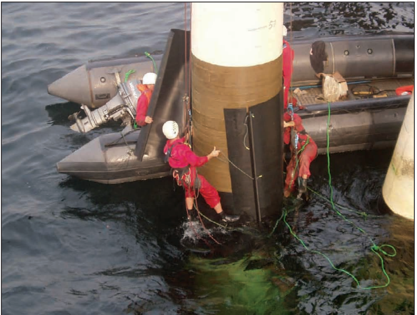
Divers fitting a 2000 FD Jacket to a 1.3m diameter pile.
