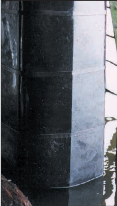
Hexagonal pile protected with SeaShield Series 100 system.
