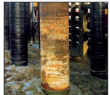
Cleaned pile ready for the application of the Seashield Series 80 System.
