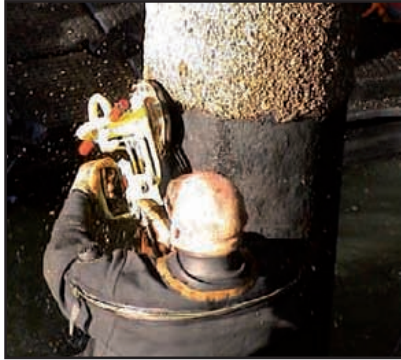
Cleaning with a power tool.
