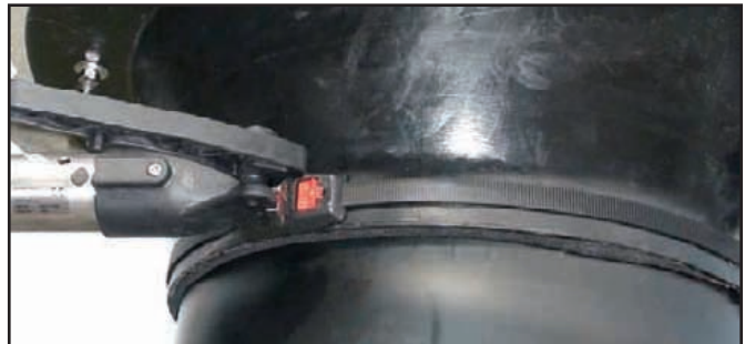
A 19mm band fixing is used to get a good seal over the existing SeaShield system.
