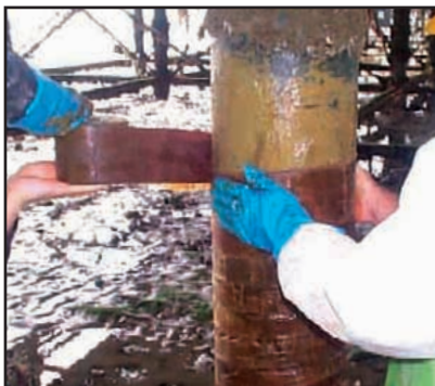
Applying Denso Marine Piling Tape.
