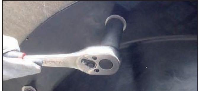
The Pile Cap is bolted to the underside of the jetty deck.
