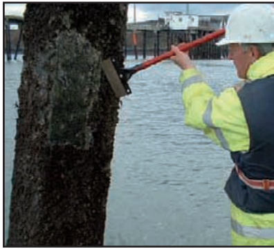
Cleaning with a hand scraper.
