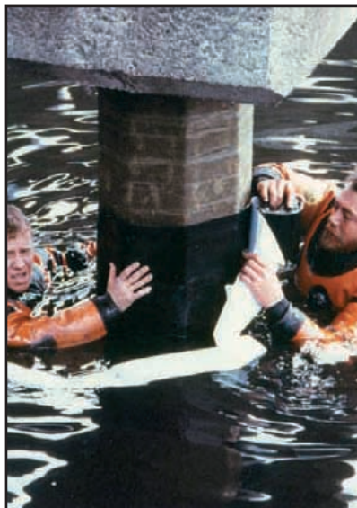
Application of Densopol 80 Marine Tape over the inner petrolatum tape layer.
