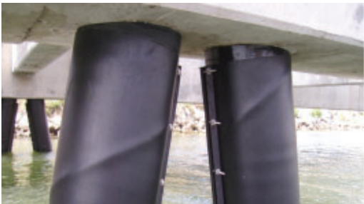
Pile protected from with Denso's SeaShield™ Series 2000HD.
