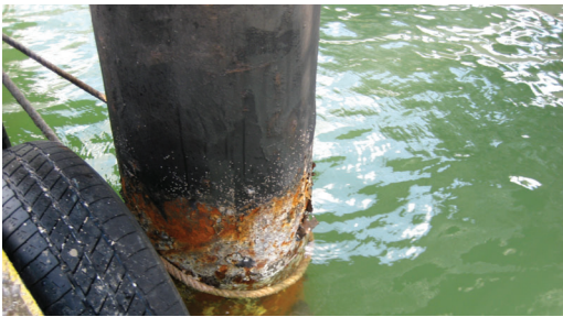
Severe corrosion of pile prior to cleaning.
