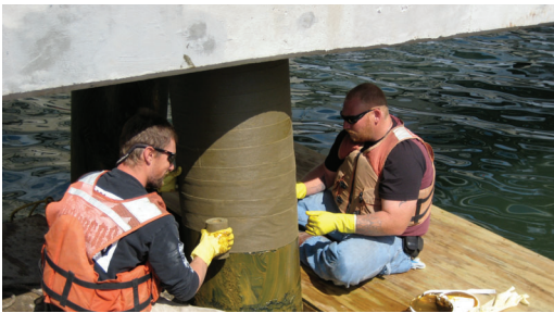
Wrapping the prepared pile with Denso Marine Piling Tape.
