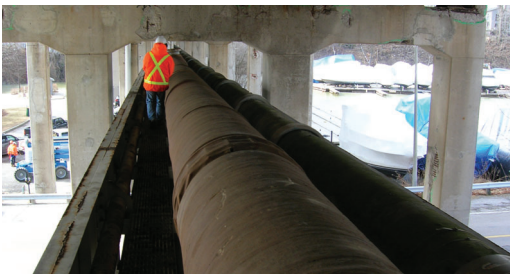
75ft. above a local parking lot the tapes were supplied and the underside applied by an operator on a lift truck.
