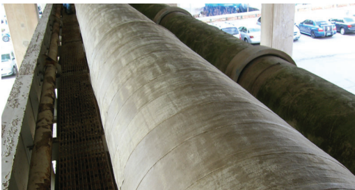
The concrete pipeline wrapped with Denso LT Tape.
