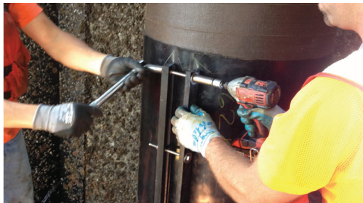
Installing the 80 mil HDPE outercover with M10 316SS fasteners.
