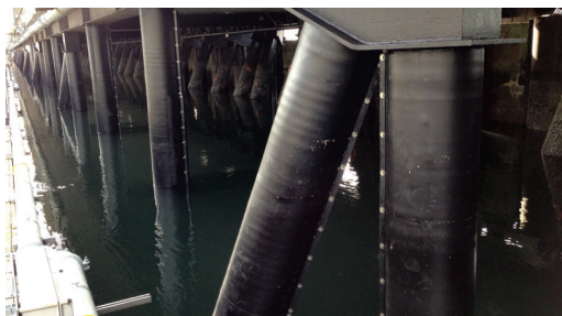
Completed piles fully protected with the SeaShield™ Series 2000HD System.
