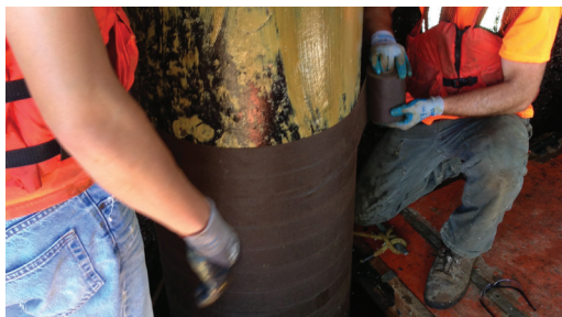
Installation of Denso S105 Paste and Densyl Tape to a 24" steel pile.
