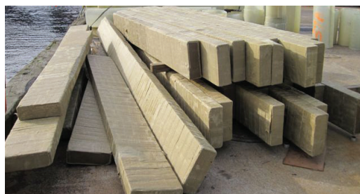
Rectangular timber headers were wrapped with Denso Petrolatum Tape.
