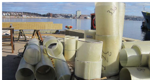
SeaShield™ 500 FRP jackets ready for installation.
