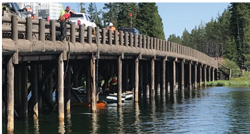
Contractor preparing deteriorated timber piles for the installation of Denso's SeaShield™ Series 500 Fiber Glass Jacket System.
