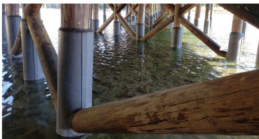
Timber piles fully protected using the SeaShield™ Series 500 System from weathering and deterioration.
