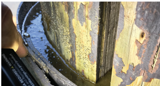
Close up of the pumpable SeaShield™ 550 Epoxy Grout within the fiber glass jacket.
