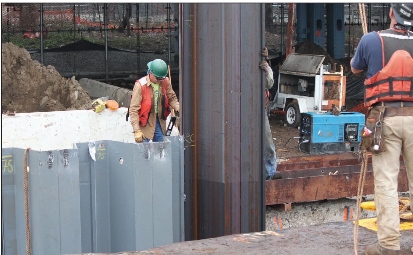
Aligning the pile as it is being driven down in place.
