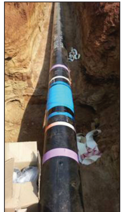
Below: The water pipeline joints protected with Denso Ultraflex 1250.
