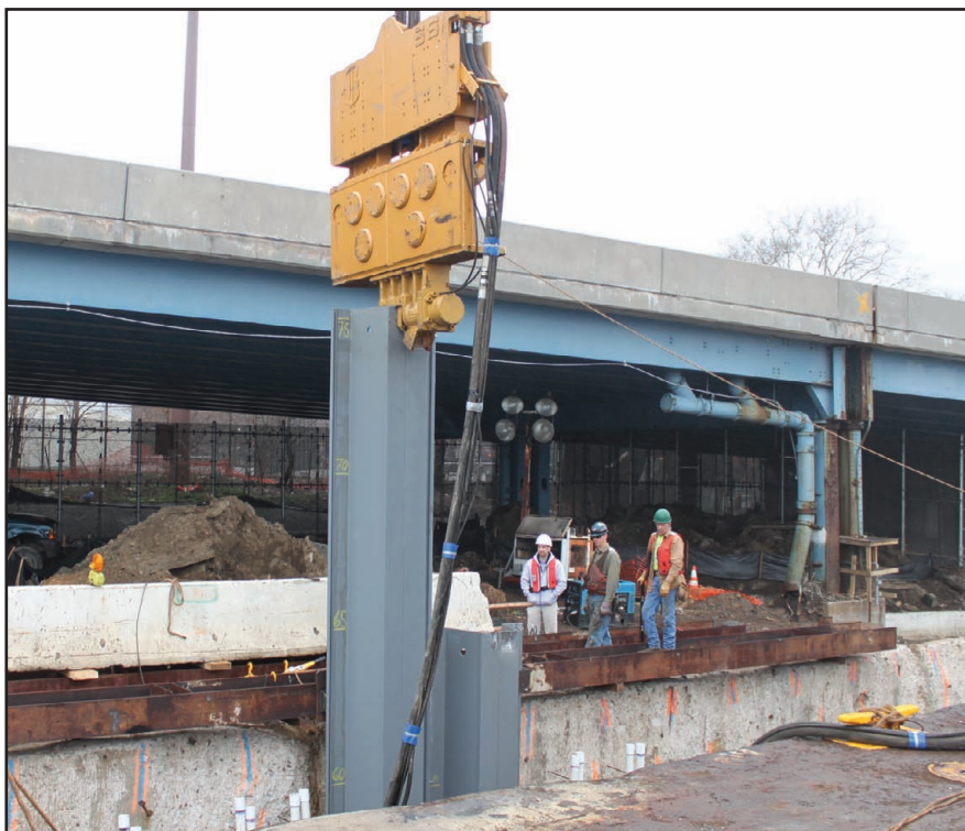
Driving the sheet piles.
