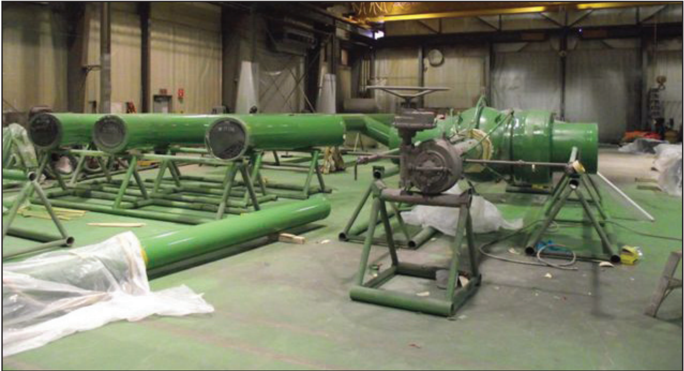
Factory coating pipelengths with Protal Liquid Epoxy.
