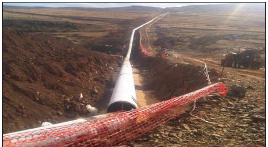
Above: The water pipeline in situ.
