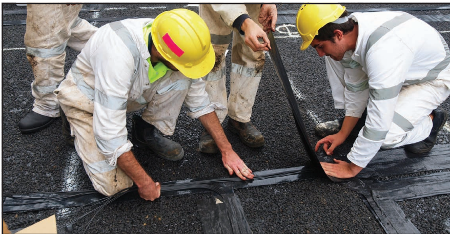
Photos above and below: Fixing the Ezyloops to the new bridge road surface.
