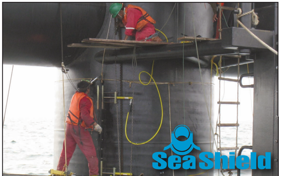
The HDPE jacket is installed, completing the SeaShield 2000FD system.
