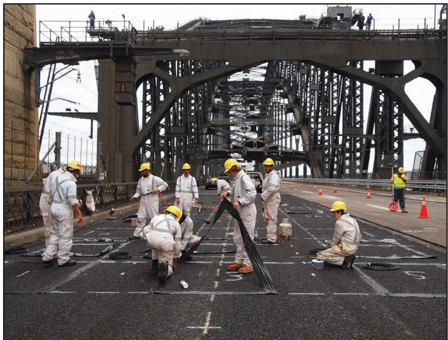
Photos above and below: Fixing the Ezyloops to the new bridge road surface.
