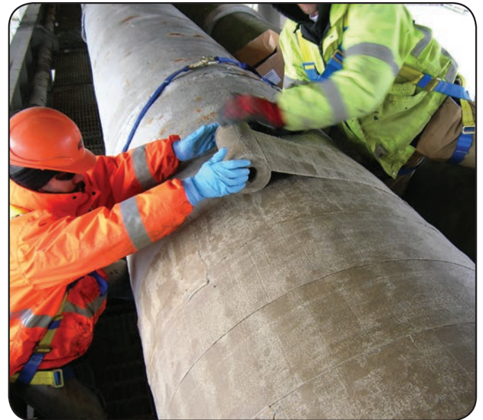
Canada - Protecting a sweating concrete water pipeline in sub zero conditions. Halton Region near Toronto.
