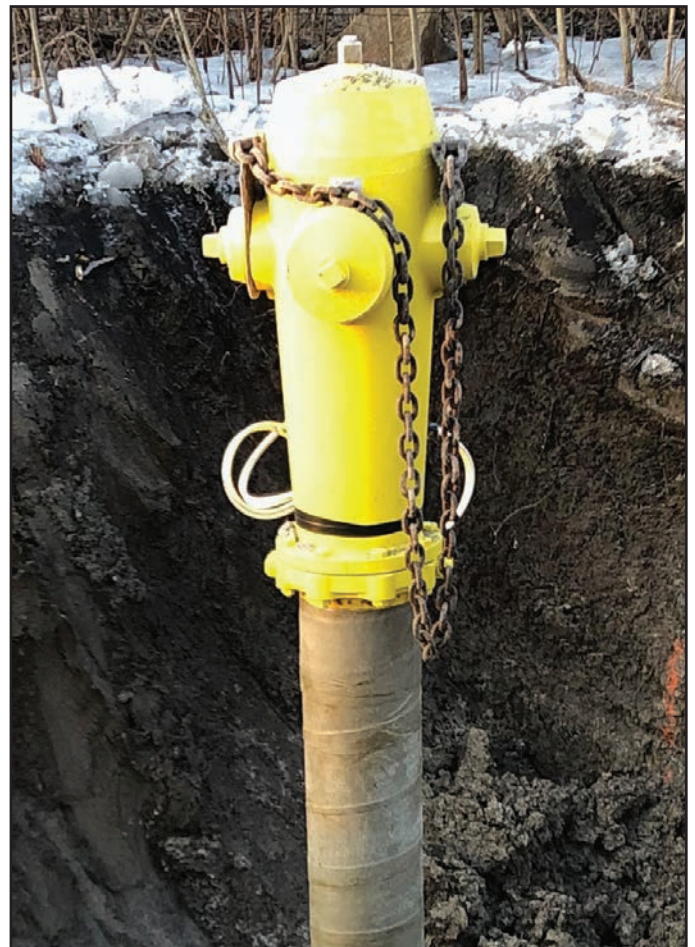
Water hydrant supply pipework protected with the Denso LT™ Petrolatum System.
