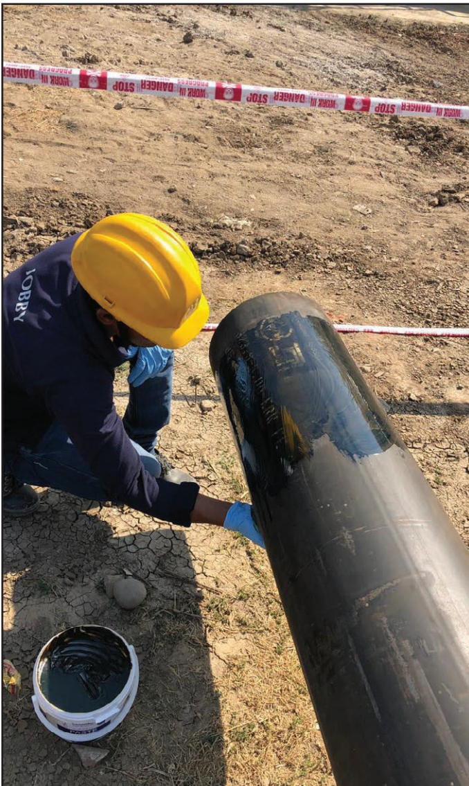
Denso Paste™ is applied to the cleaned pipe surface.
