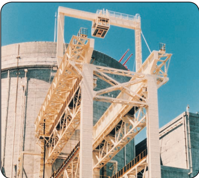
South Africa - 30 years of proven, maintenance-free, protection of a huge gantry crane situated in a highly corrosive coastal environment - as part of the Denso Steelcoat™ Systems.
