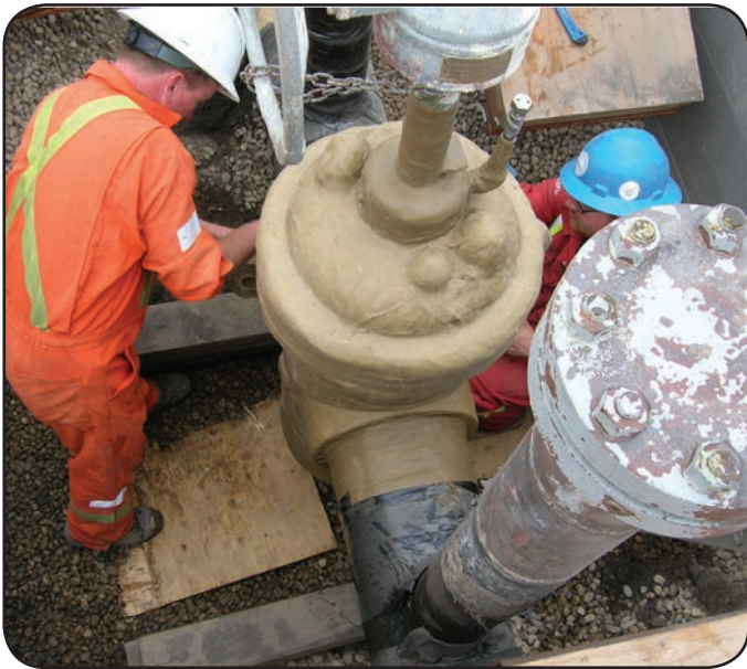
Canada - Protecting buried petroleum pipeline valves for the Sun-Canadian joint venture in Southern Ontario.
