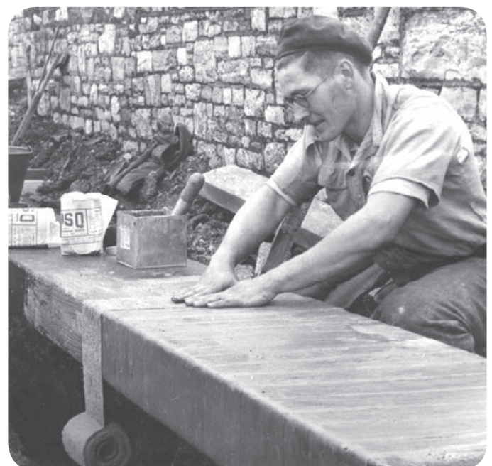
Protecting steel beams.
