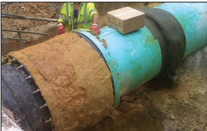
Denso Profiling Mastic™ is used to create a smooth profile prior to tape wrapping.
