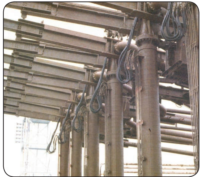
UK - Protecting loading booms at the Esso Milford Haven Refinery, using weatherboard and spiral tape wrapping techniques.
