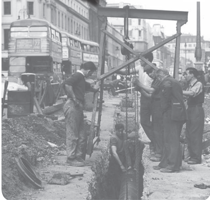
A pipeline is replaced during the rebuilding of London in the 1950's.
