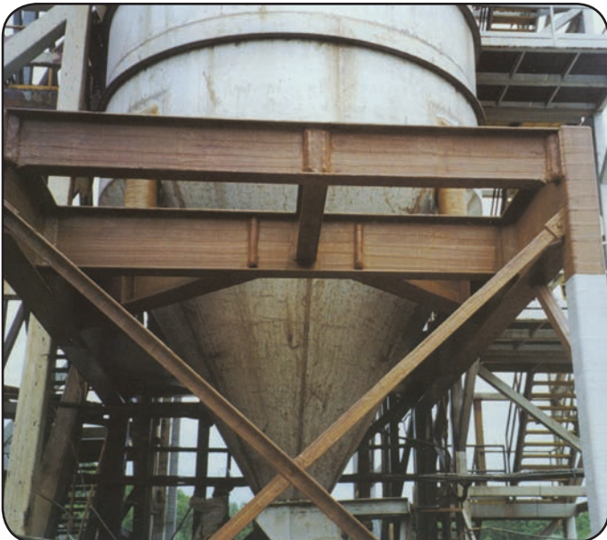
USA - Protecting parts of the steel headframe in the severe corrosive environment of a salt mine at the Cargill Salt Facility, Avery Island, Louisiana.
