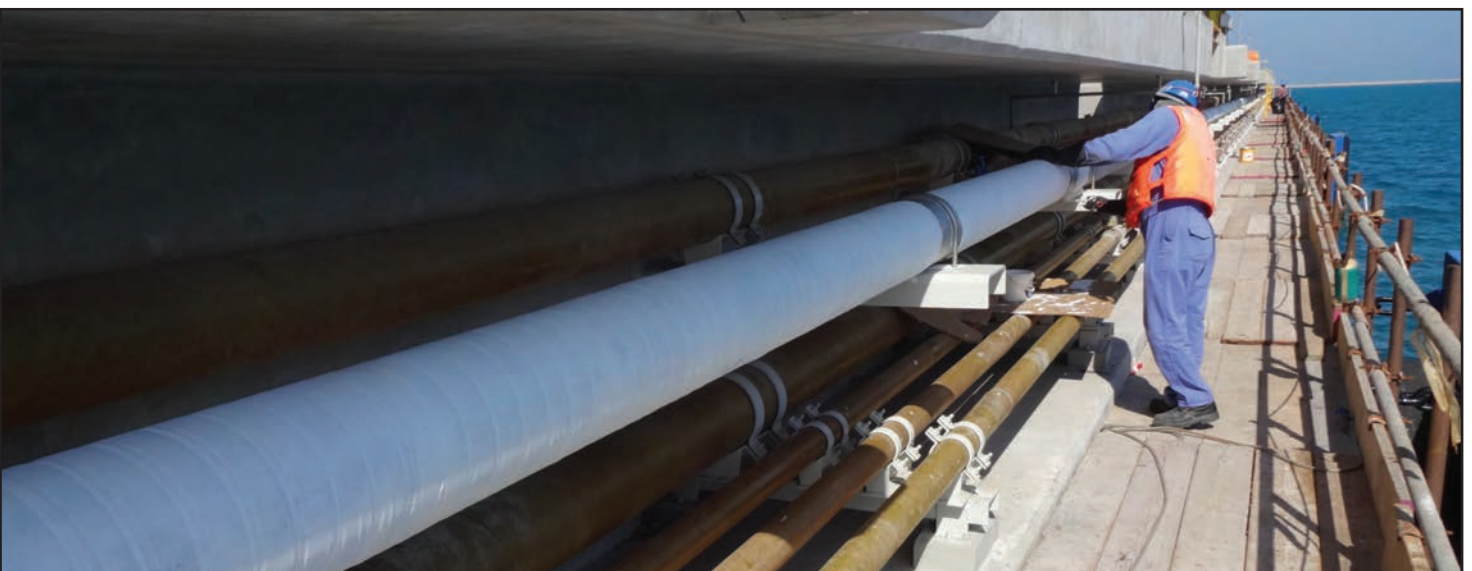
After applying a spiral wrap of Denso Ultraseal RT™ Tape, two coats of Denso Acrylic Topcoat™ completes the pipe protection system.
