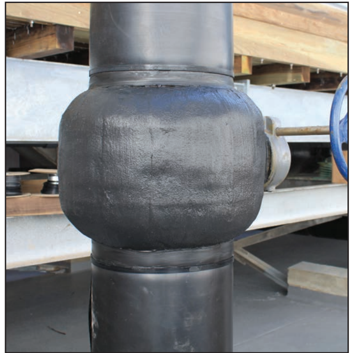
Archco 15™ Acrylic Topcoat is brush applied onto Densyl™ Tape protecting a valve flange as a top coat.
