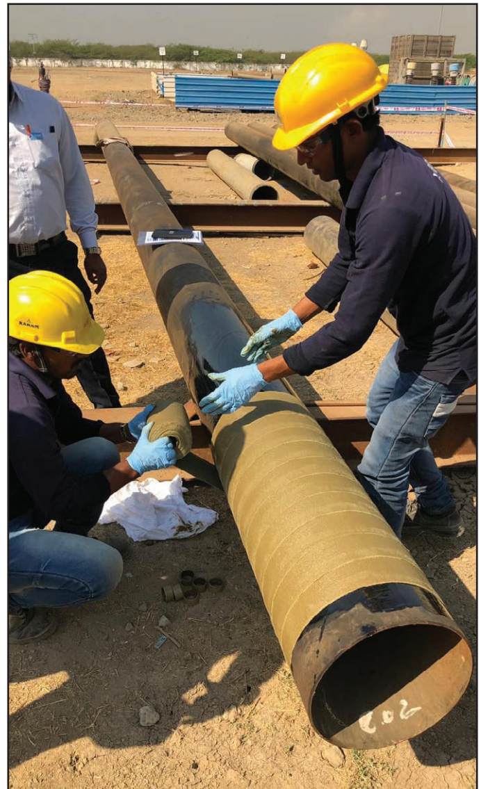
Densyl™ Petrolatum Tape is circumferentially applied over the Denso Paste™.
