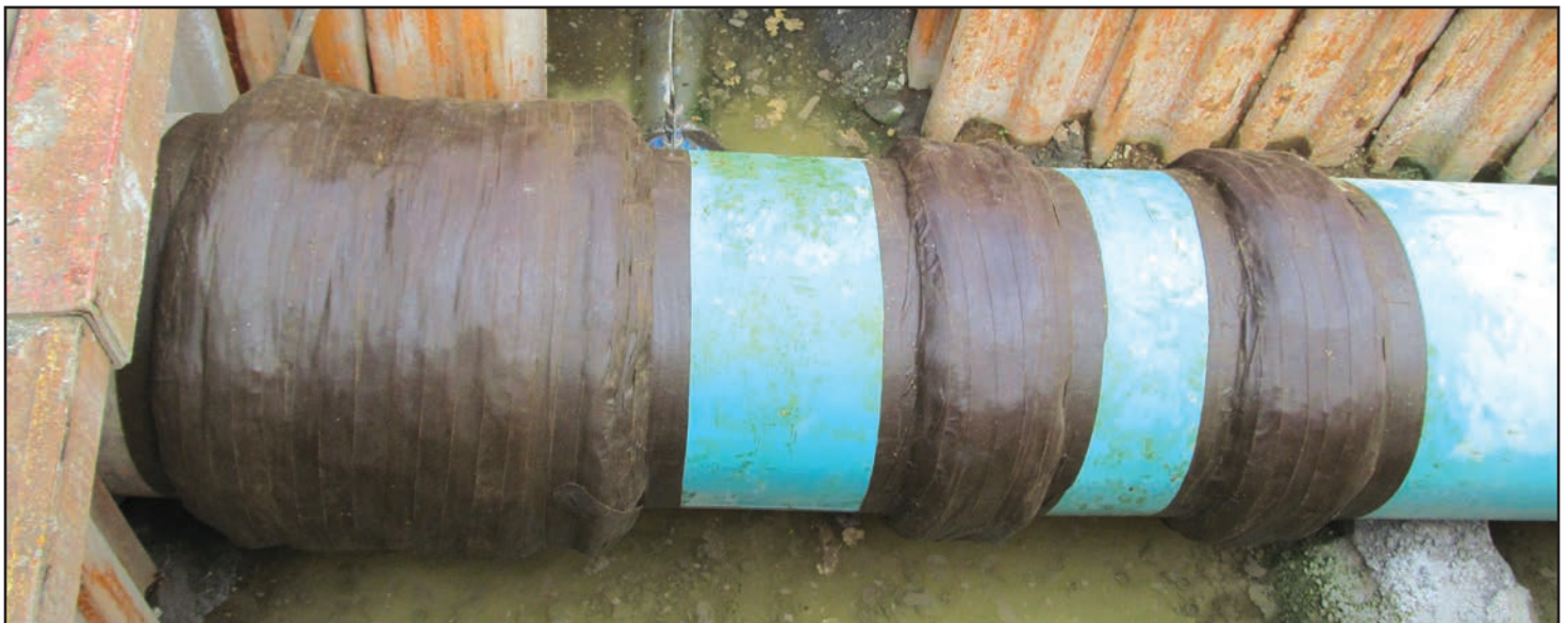
The completed Denso™ Petrolatum Tape System protecting the pipe joints.
