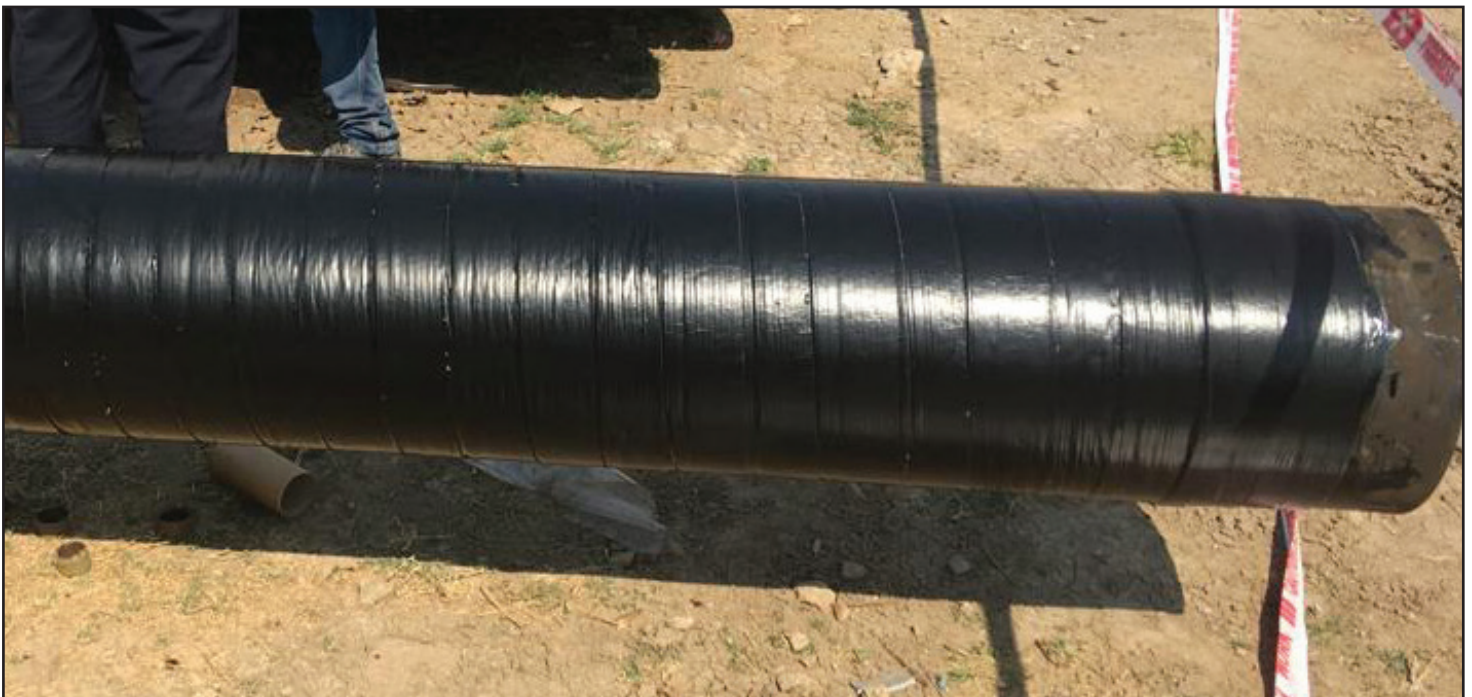
A completed section of pipe.
