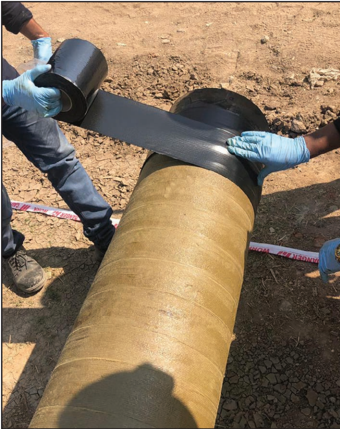
A wrap of Densopol 60HT™ Tape is applied to complete the system.
