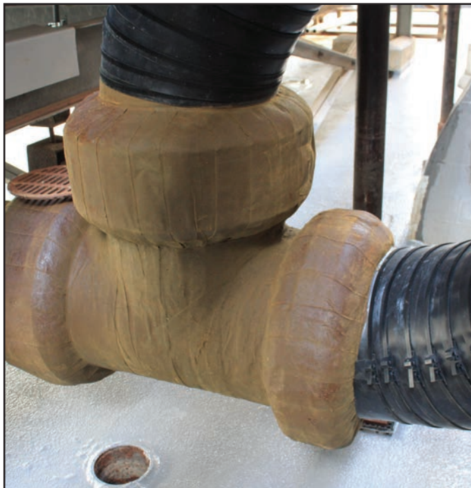
A large pipe tee joint wrapped with Densyl™ Tape prior to the application of Archco 15™ Acrylic Topcoat. The Denso HDPE Outerwrap™ is shown on the connected pipes.
