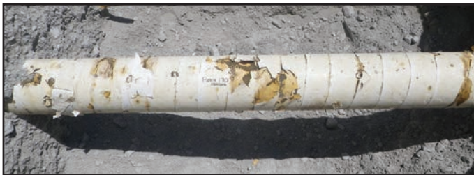
The original Denso™ system had probably been damaged by backfill.
