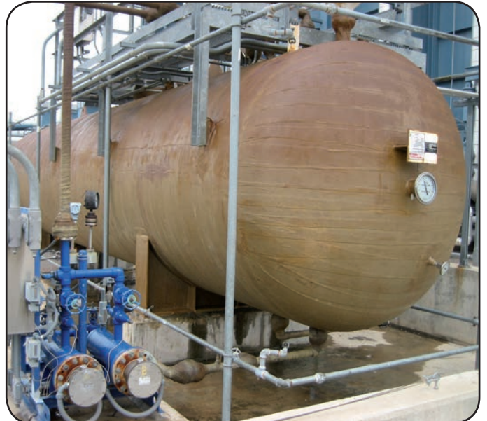
USA - Protecting constantly sweating steel ammonia tanks at the Lower Colorado River Authority (LCRA) Bastrop facility, Texas.
