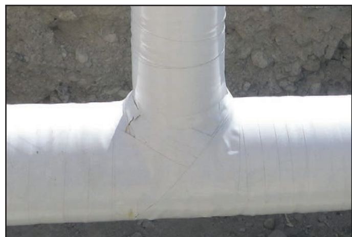
The new tie-in protected with the the Denso™ Petrolatum Tape System.
