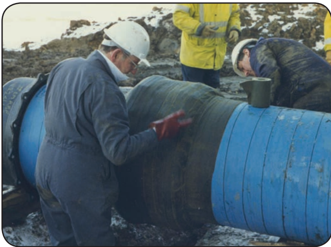
UK - Protecting buried Viking Johnson Couplings on water pipework at Whorely Reservoir which supplies Darlington and parts of Teeside.
