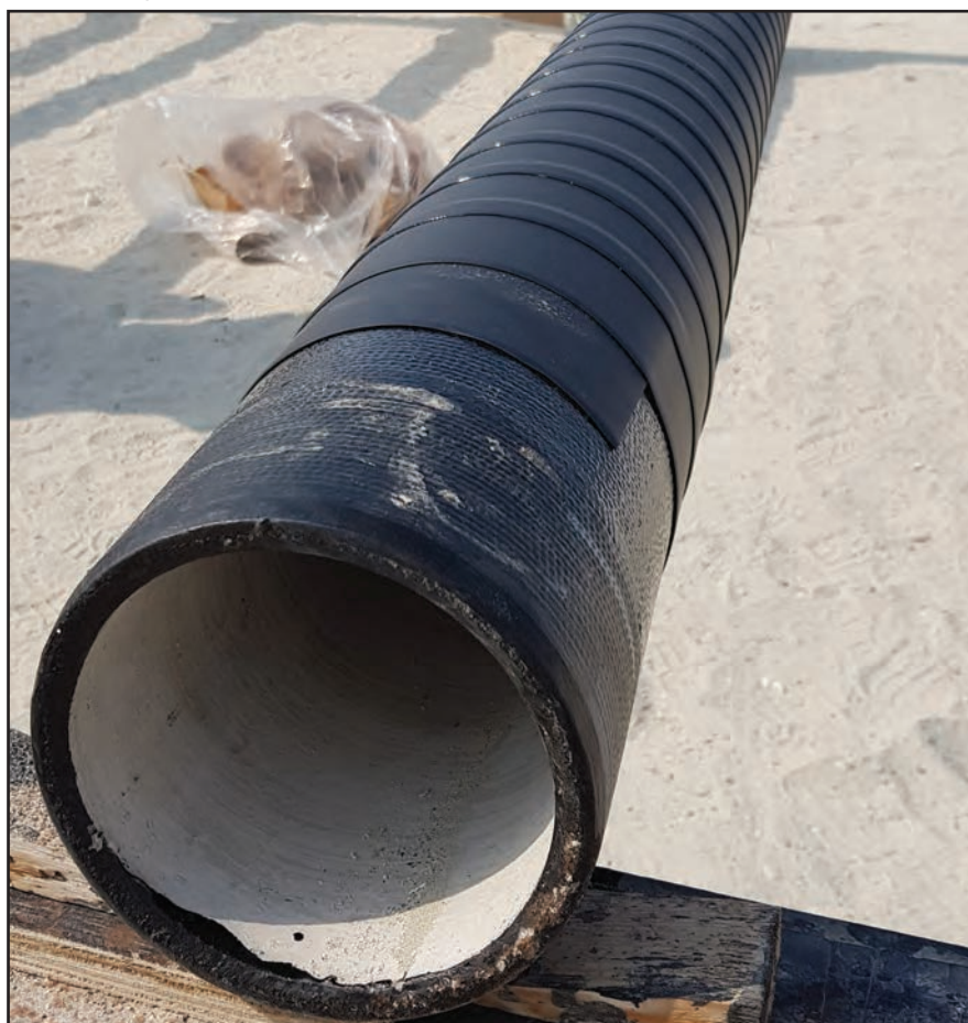
The pipe lengths were wrapped prior to installation.
