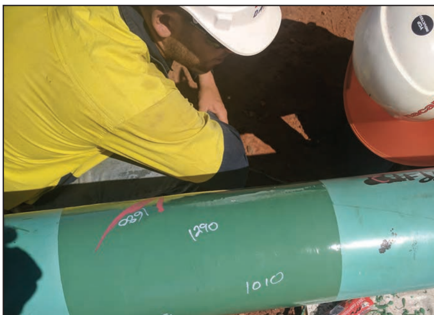
Application of Denso Protal 7200™ to a gas pipeline field joint.
