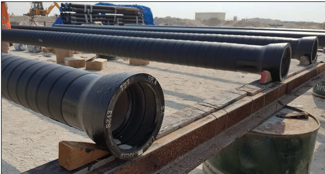
The pipe lengths were wrapped prior to installation.
