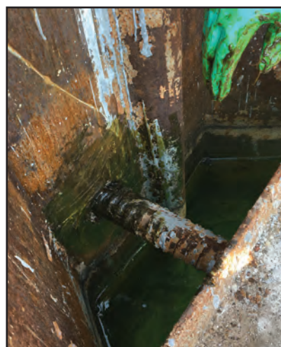
One of the anchor rods passing through the sheet piling.
