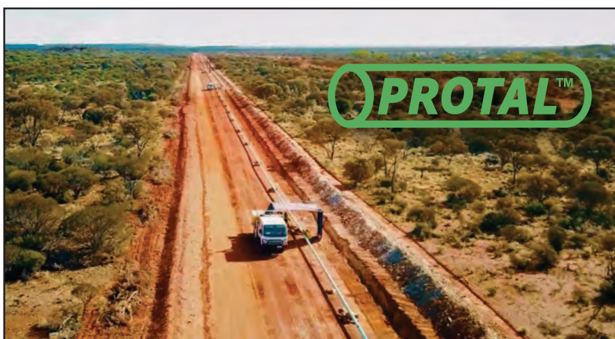
The installation of the new gas pipeline underway.
