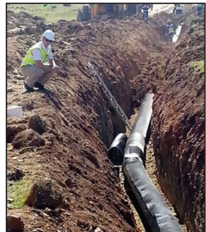
Inspection of field joint repair and securing of the Denso Stoneguard.
