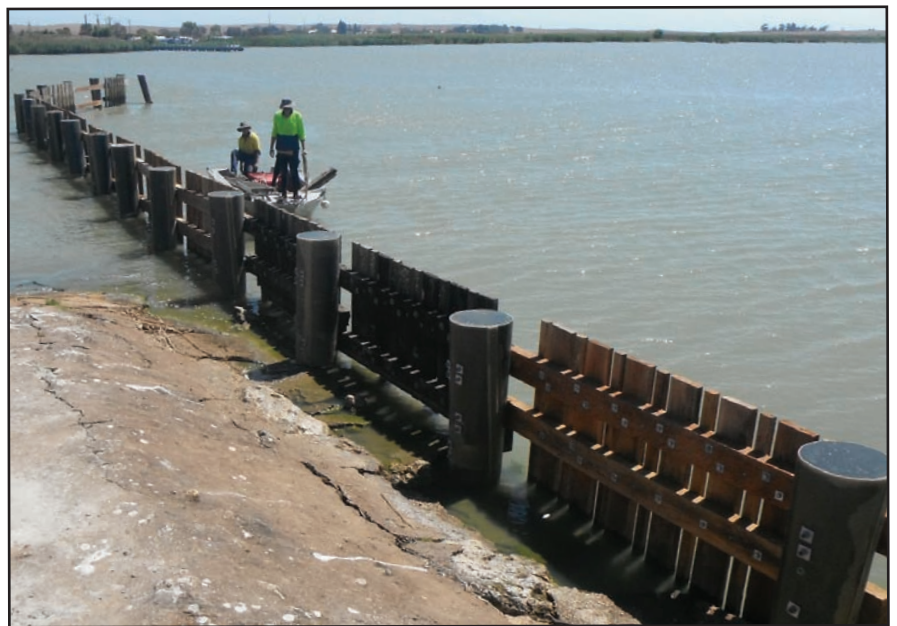
The wave screen with SeaShield Series 500 system installed on the timber piles.
