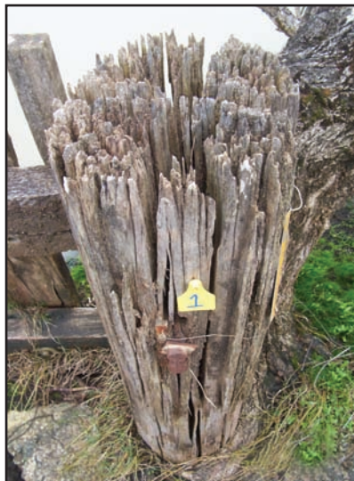
A close up of one of the eroded timber piles.
