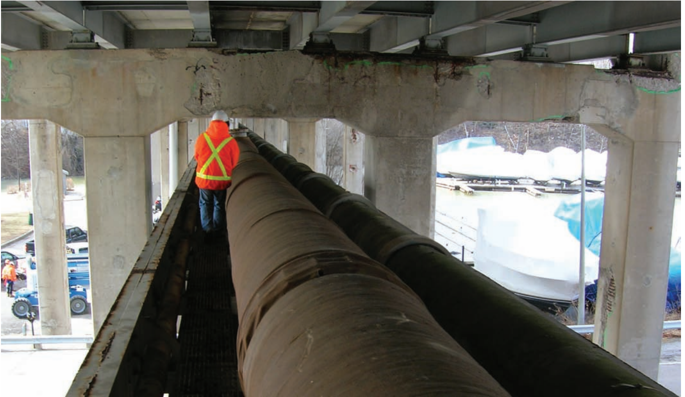
The concrete pipeline wrapped with Denso LT Tape.
