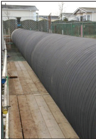
Above: Torskey pipebridge and below Fallingworth protected with the Denso Steelcoat 400 system.
