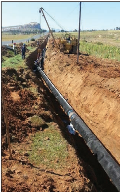
Sidebooms laying the 660mm dia Denso Stoneguard wrapped pipe prior to installation.
