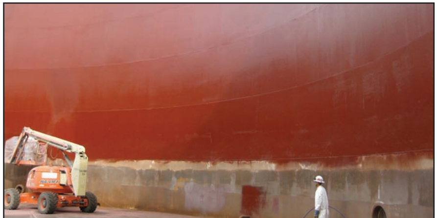
Below: The open top tank side walls were primed with Archco 400 (red).
