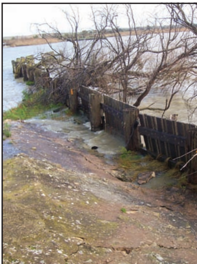
The badly dilapidated wave screen.
