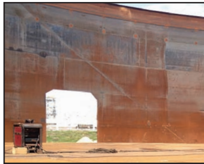
Below: The open top tank side walls were primed with Archco 400 (red).
