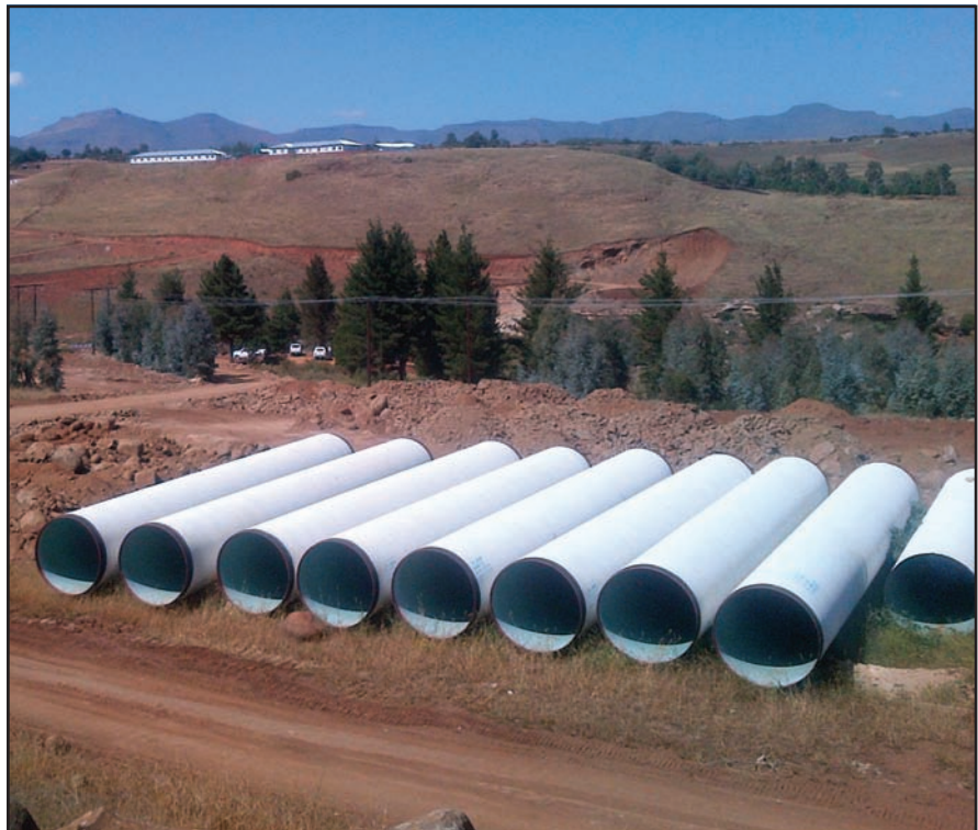
The 1100mm dia Bituguard coated pipe for the transport of water from the Metolong Dam to the water treatment plant, with a view of the Maluti Mountains in the background.
