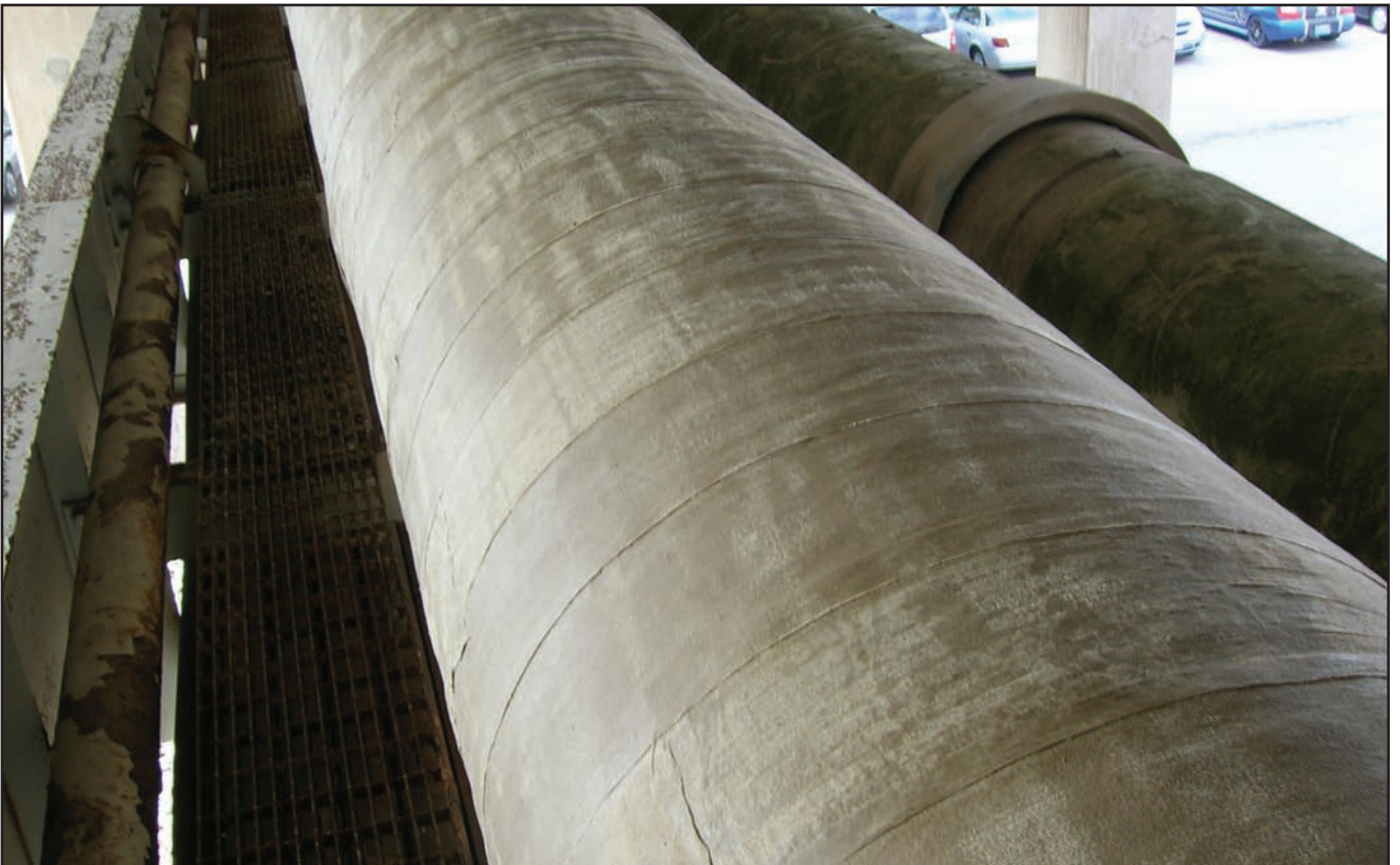
The concrete pipeline wrapped with Denso LT Tape.
