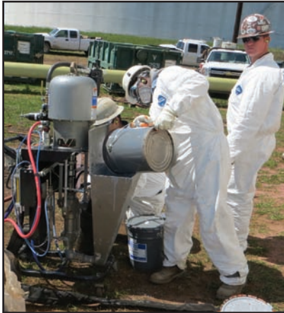
Getting the spray unit ready with Denso's Archco-Rigidon Tank Lining coating.
