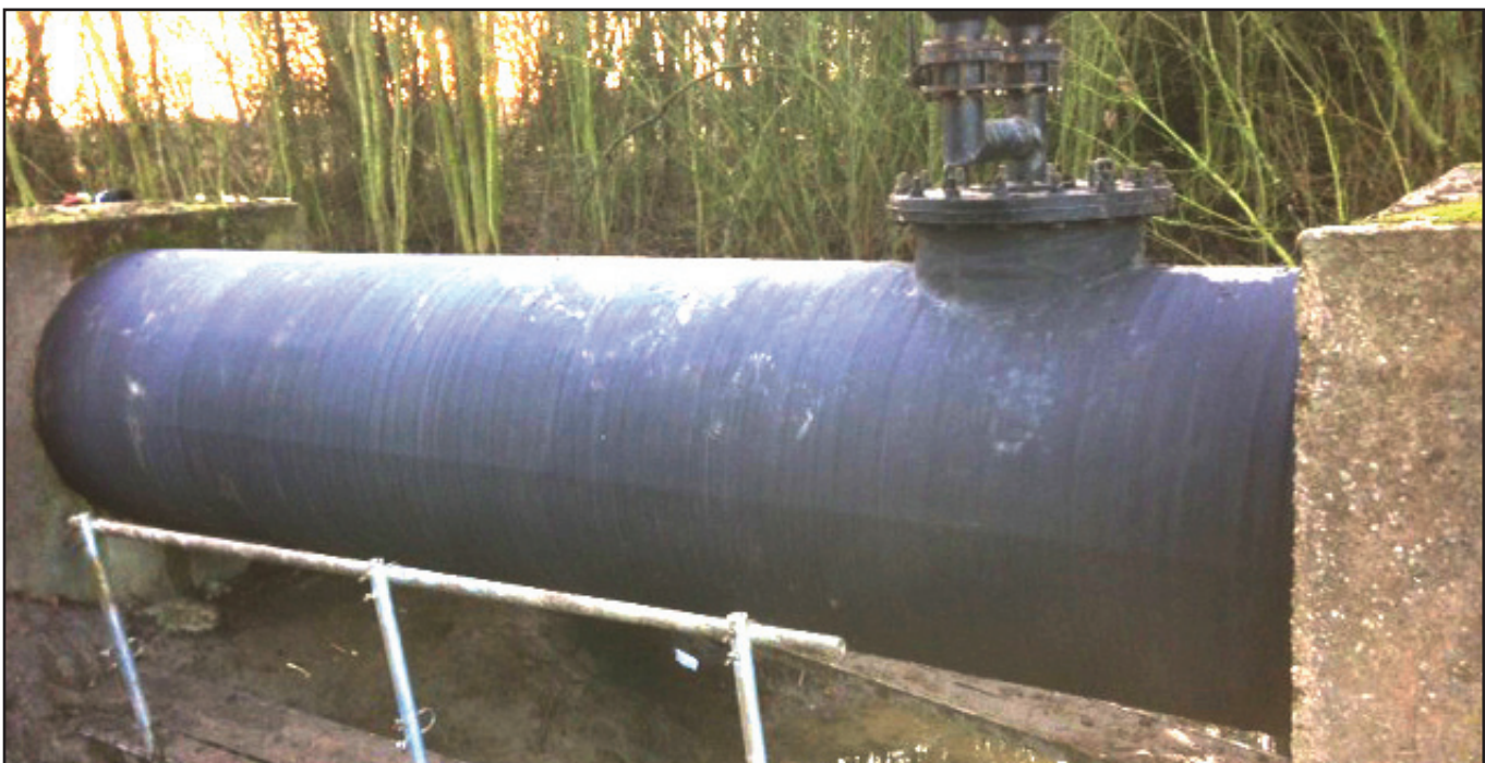
Above: Torskey pipebridge and below Fallingworth protected with the Denso Steelcoat 400 system.
