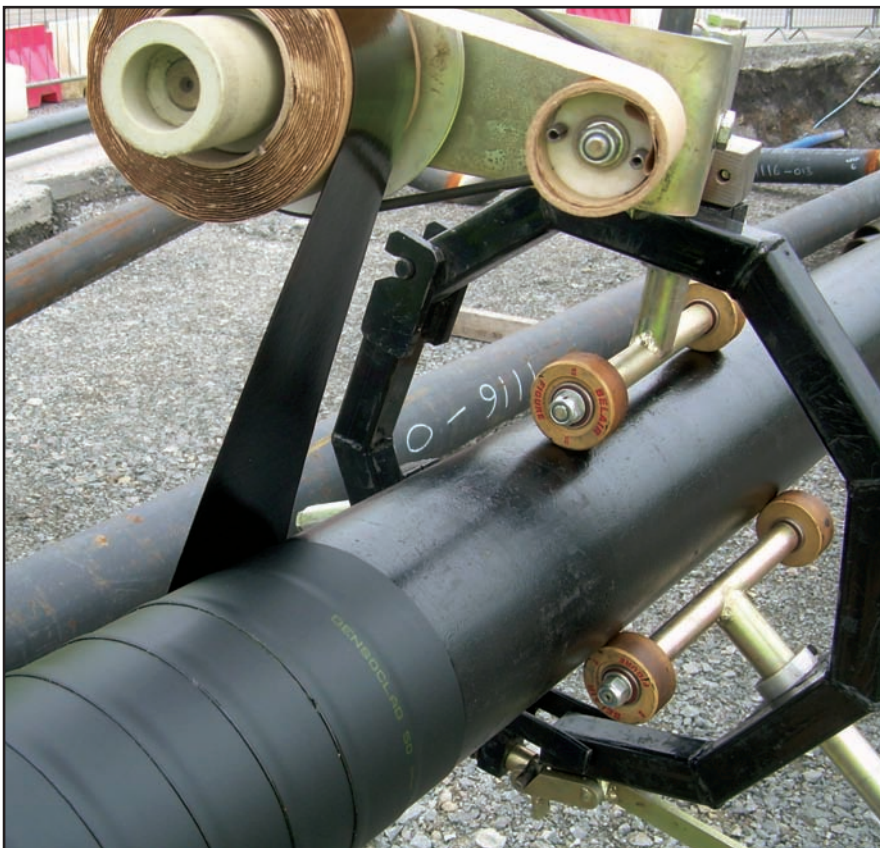
Above: The new Scrabster Quay pipework was wrapped with Densoclad 50 Tape.
