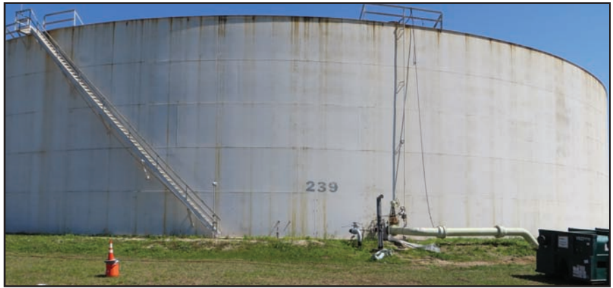
Below: Internal tank walls corroded and in desperate need of a Archco System.
