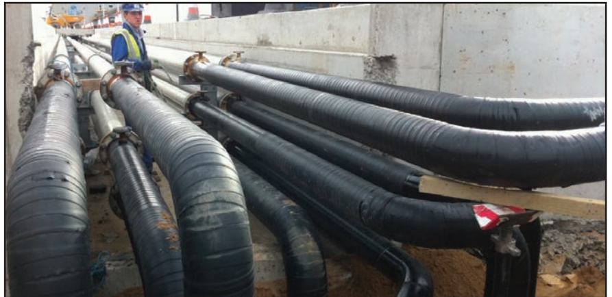
Above: The new Scrabster Quay pipework was wrapped with Densoclad 50 Tape.
