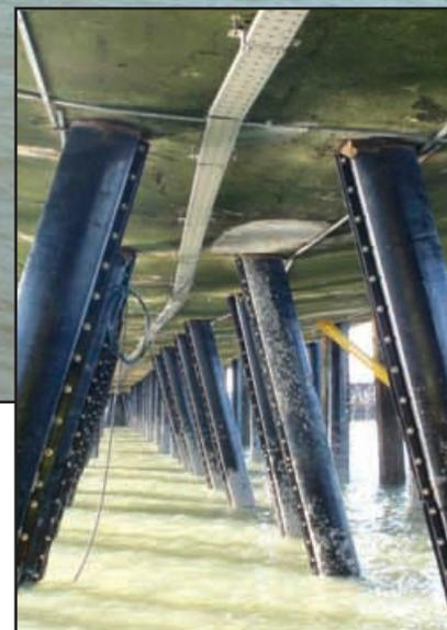
A Denso SeaShield system was again chosen to protect the new independent fender piles as well as the existing piles from the corrosive marine environment. This can be a major problem in splash zones, inter-tidal and subsea environments and the difficult area where the jetty pile meets the jetty platform.
