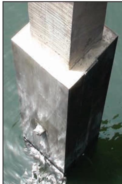
The Seashield Epoxy Grout fills the annulus between the pile and the SeaShield Jacket.
