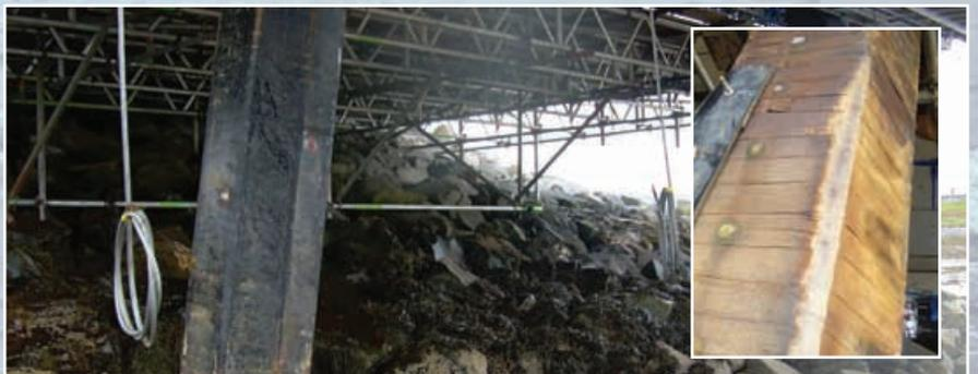
Above: The Kyle of Tongue Bridge in Scotland - inset shows close up of the excellent condition of the Denso Marine Piling Tape revealed upon jacket removal for inspection, after 22 years service.
