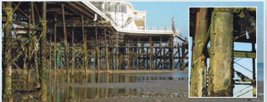
Above: Worthing Pier, Sussex - inset shows heavy marine growth cleaned off of a SeaShield jacket revealing it to be in good condition underneath and perfect working order after 27 years in service.
