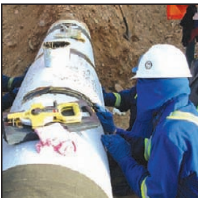
Fig 2. The Denso coatings are applied.
