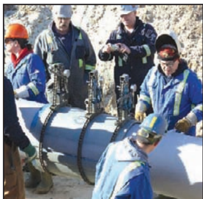
Fig 1. installation of a steel sleeve.
