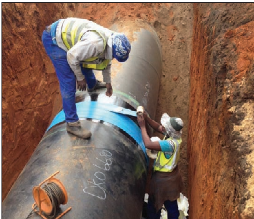
After application of Denso Primer D the joints are overwrapped with Denso Ultraflex 1250 Tape.
