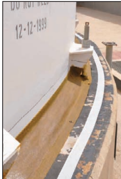
Applying the Denso Hi-Tack Tape.
