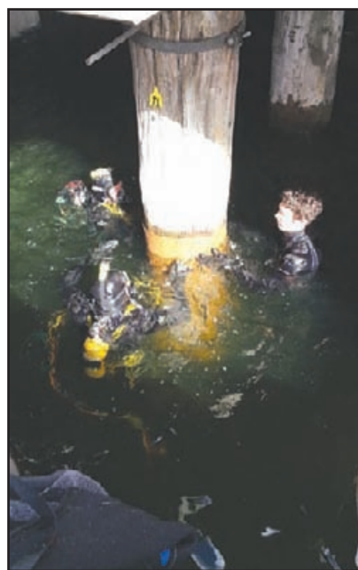
Above: Application of Denso Marine Piling Tape.
