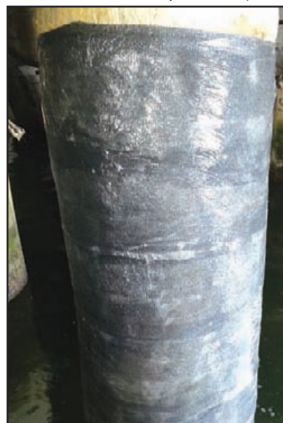
Below: The SeaShield 70 System is completed.
