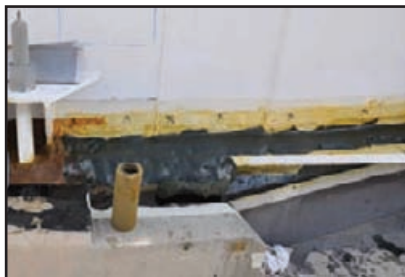
Applying the Denso Hi-Tack Primer.
