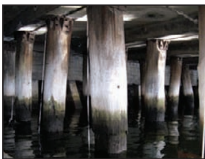
View of the timber piles beneath the dock.
