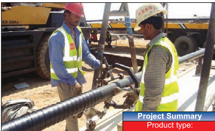
Machine wrapping the tie rods with Densopol 60HT Tape.
