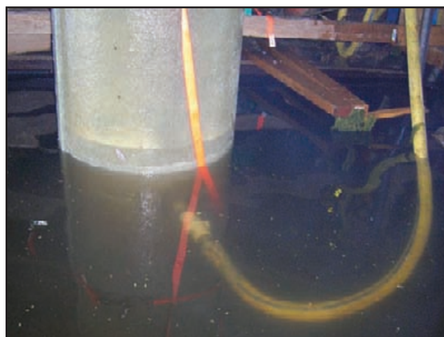
The SeaShield 550 Grout is pumped into the SeaShield 500 forms.
