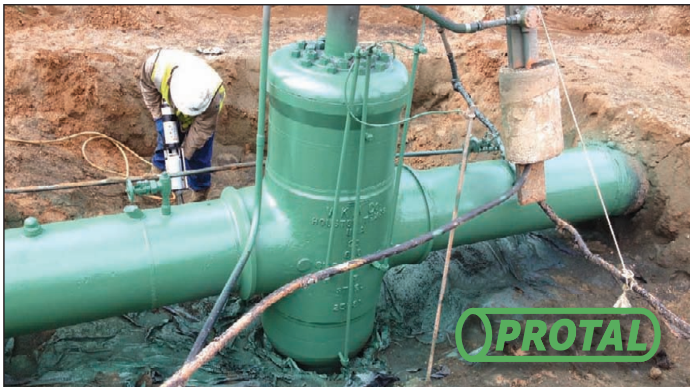
Above: Spray application of a 20" in service gate valve.
