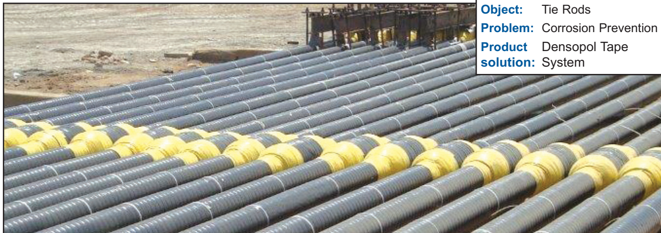
Machine wrapping the tie rods with Densopol 60HT Tape.
