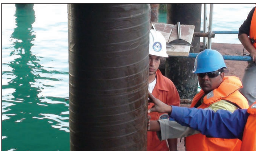
Denso SeaShield 2000 FD application begins with a circumferential wrap of Denso Marine Piling Tape to the previously cleaned pile surface.
