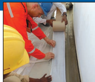
5. The Denso Ultraseal RT Tape is applied in weatherboard style.
