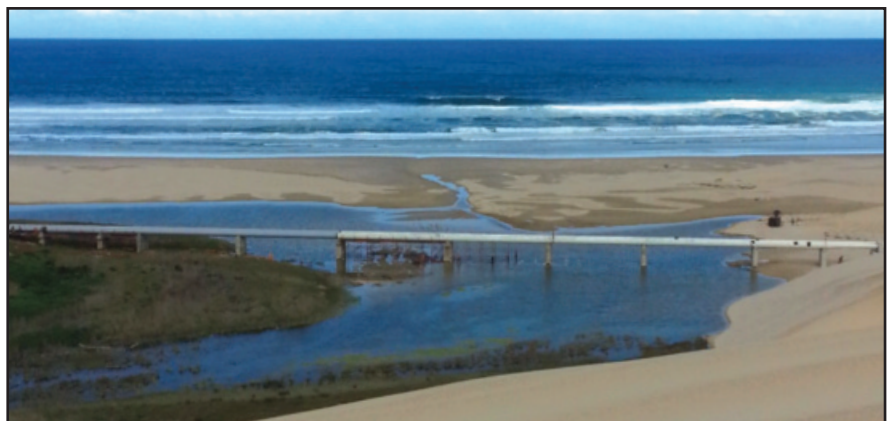
A view from a nearby sand dune shows exactly how close to the ocean the pipebridge is and the harsh environmental conditions the Denso Steelcoat 500 System needs to perform under.
