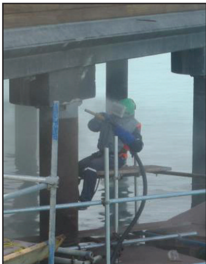
Abrasive blast cleaning of the top of the pile area to be coated with Denso Rigspray.
