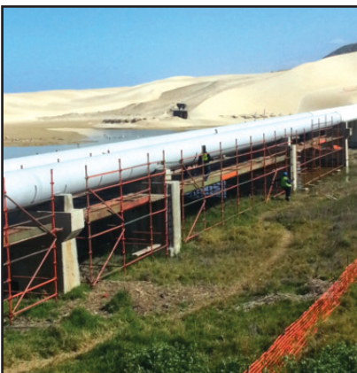
Application of the Steelcoat System progressing along the pipebridge
