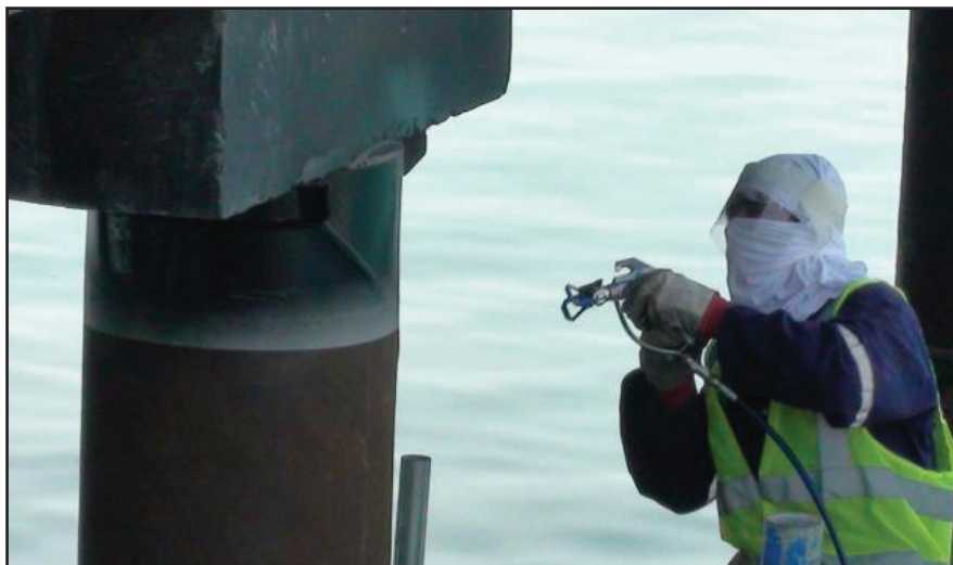
Denso Rigspray was applied by spray in two coats to a total thickness of 1200 microns.
