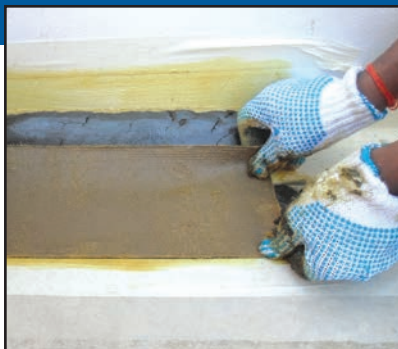
3. A layer of Denso Hi-Tack Tape is applied.
