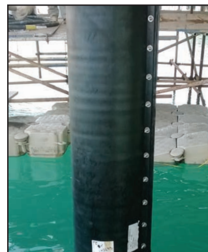
Denso SeaShield 2000 FD application begins with a circumferential wrap of Denso Marine Piling Tape to the previously cleaned pile surface.
