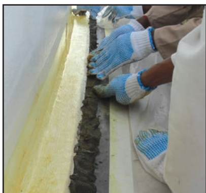
2. All voids are filled with Densyl Mastic.
