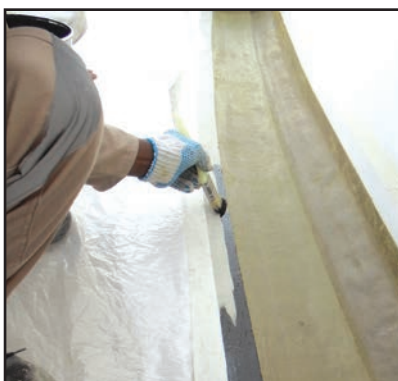
4. Denso Primer D is applied to a masked area before the application of Denso Ultraseal RT Tape.
