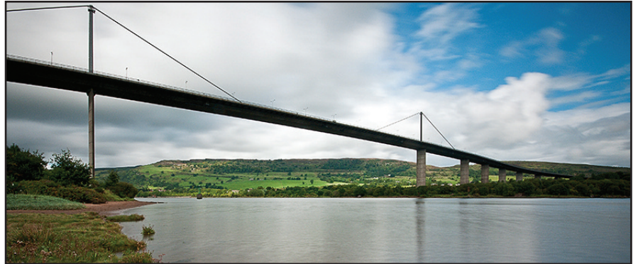
The Erskine Bridge
