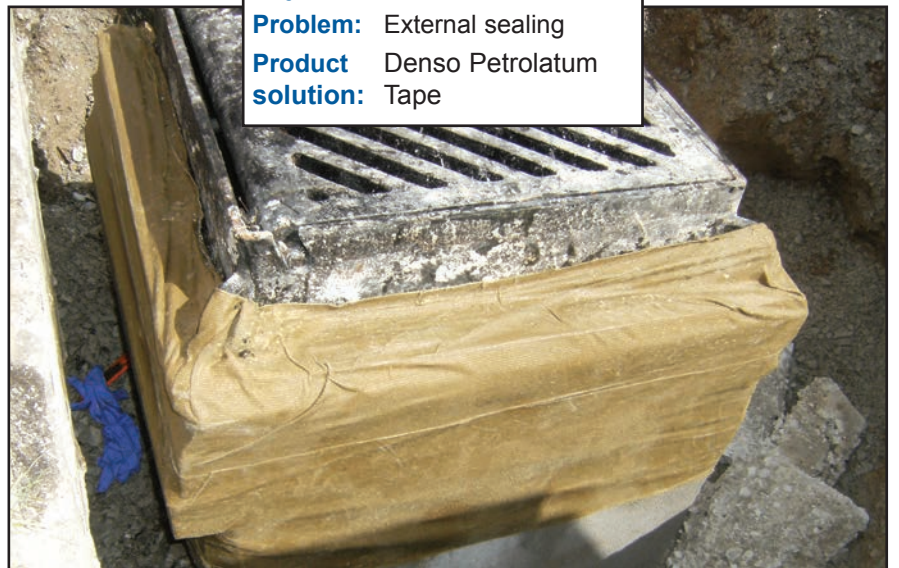
A manhole chamber in Barrie Ontario is exposed for repair is wrapped with Denso Tape.
