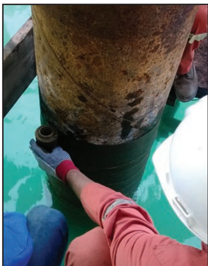
Denso SeaShield 2000 FD application begins with a circumferential wrap of Denso Marine Piling Tape to the previously cleaned pile surface.
