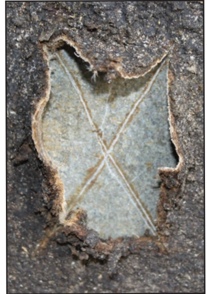
The removal of a small patch of the Denso Tape coating for an inspection of one of the support I-Beams reveals the steel to be in excellent condition after 37 years.
