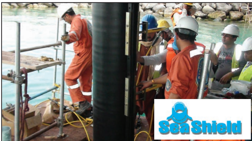
The SeaShield 2000 FD Jackets are then placed over the pile and bolted together to complete the system.
