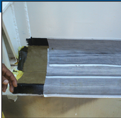
3. The Denso Ultraseal RT Tape is applied in weatherboard style
