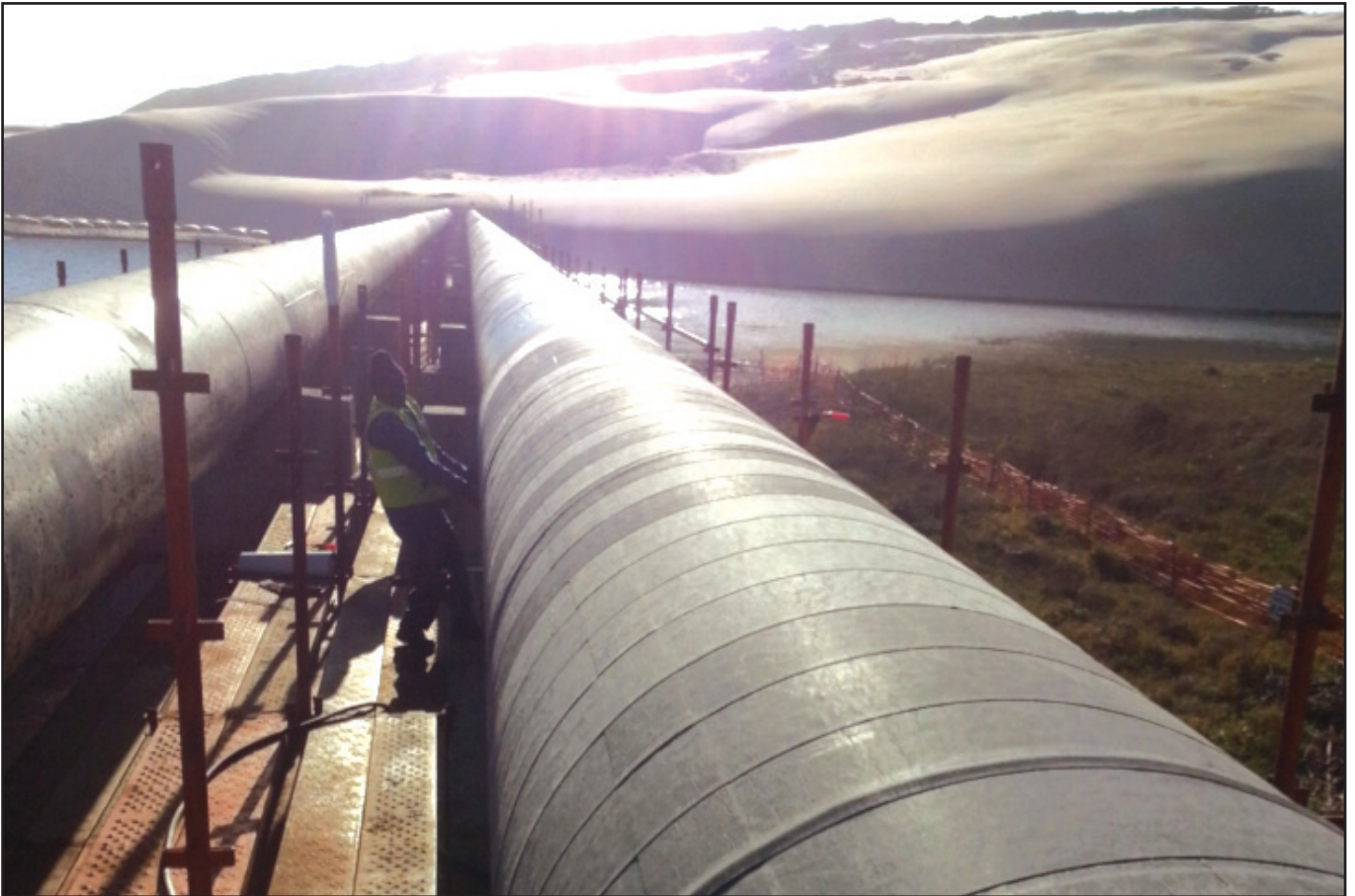
Application of the new Denso Steelcoat 500 system.
