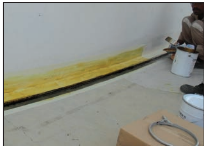
1. After cleaning the vulnerable area is primed with Denso Hi-Tack Primer.
