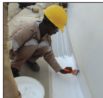
6. A coat of Denso Acrylic Topcoat is applied over the Denso Ultraseal RT Tape.
