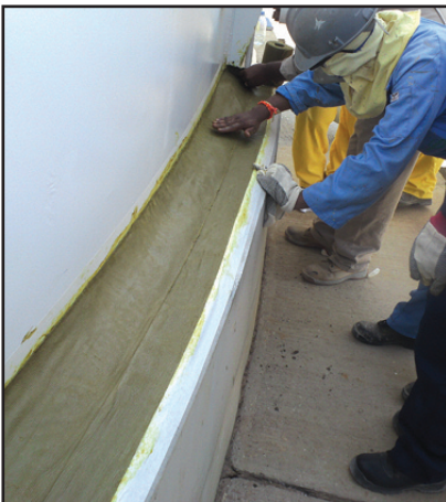
1. After cleaning and then priming with Denso Hi-Tack Primer the Denso Hi-Tack Tape is applied.
