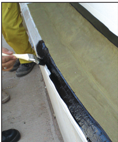
2. Denso Primer D is applied to the masked area before the application of the Ultraseal RT Tape.
