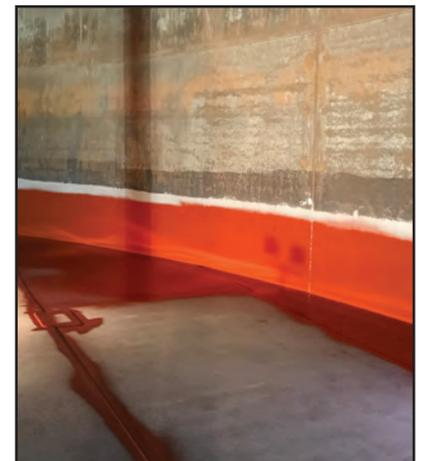
Archco 400 primer being applied to the blasted floor and side walls of the tank.
