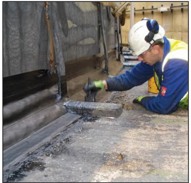
Above and below: After a single layer of Denso Ultraseal RT Tape is applied, a coat of Denso Topcoat completes the Steelcoat system application.
