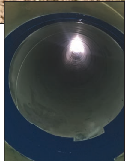
Above: Internal field joints lined with the epoxy Denso ST100 System.
