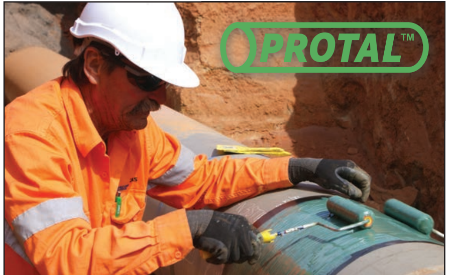
Above & below: Denso Protal 7200 being applied to protect the gas main field joints.
