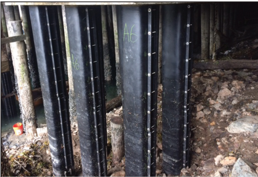
Completed H-Piles fully protected with the SeaShield Series 2000HD System.
