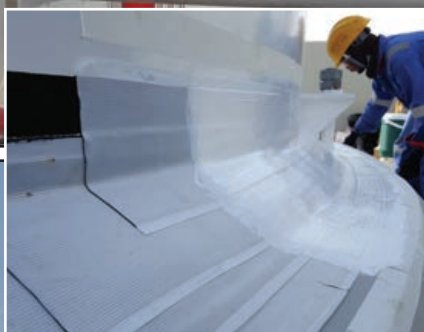
Above: Denso Acrylic Topcoat is applied over the layer of Denso Ultraseal RT.
