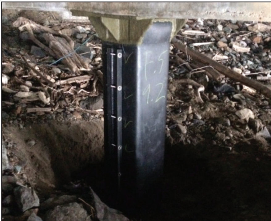
Above: Pile cap/gusset area protected with the SeaShield SplashZone UW Epoxy.
