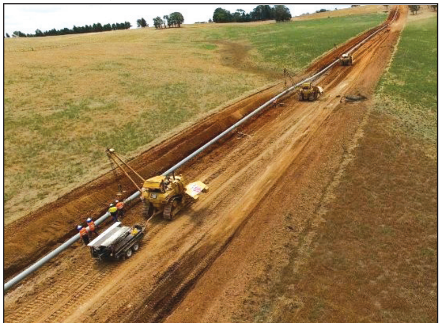
A section of the new gas main under construction.
