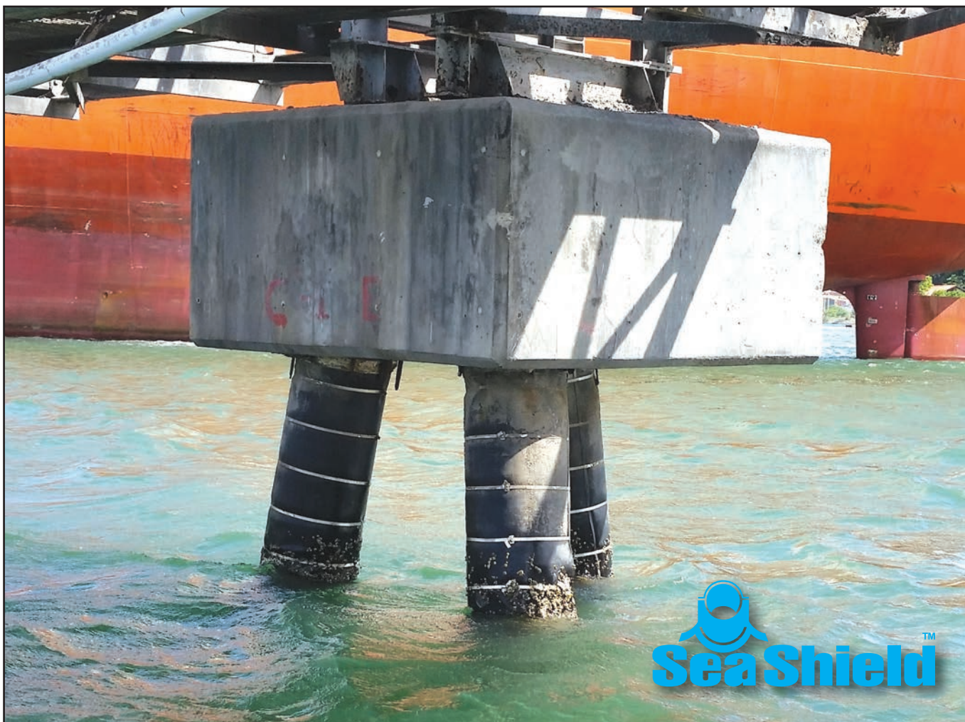
Below: The original SeaShield 100 application from 1999 still good and showing the expected amount of marine growth after 18 years.
