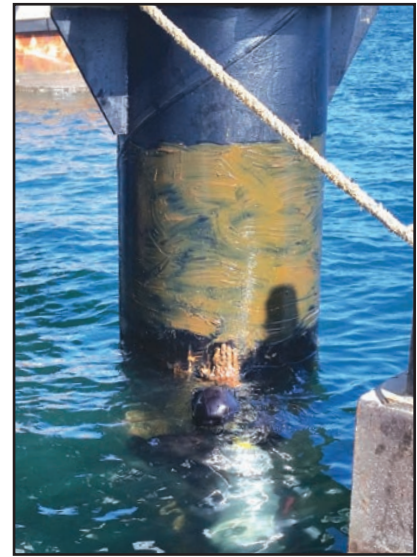
Above: After cleaning, the Petrolatum Paste is applied to the pile.
