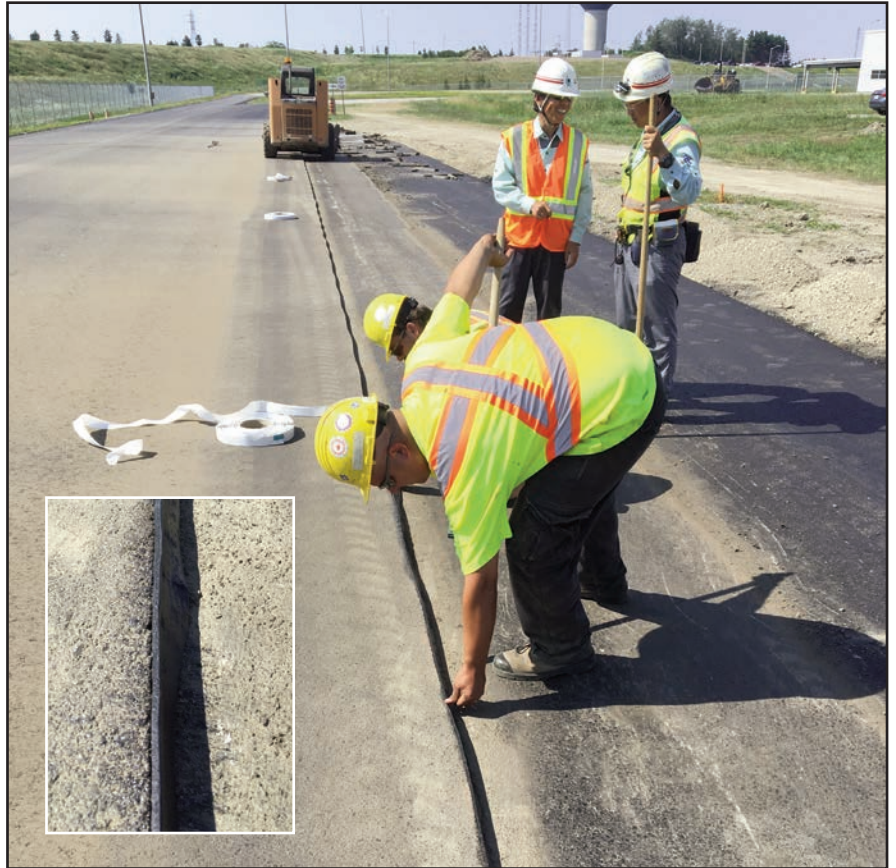
Above: After first priming, the Densoband rubber bitumen flexible jointing strip is laid along the vertical face of the joint.
