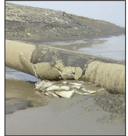
The damaged concrete pipeline coating.
