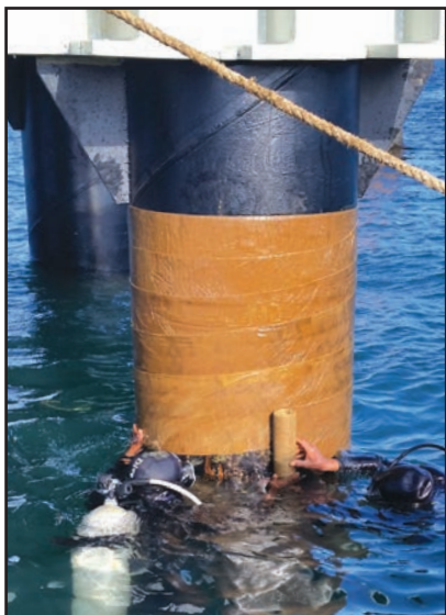
Above: The Petrolatum Tape is then applied over the Paste.
