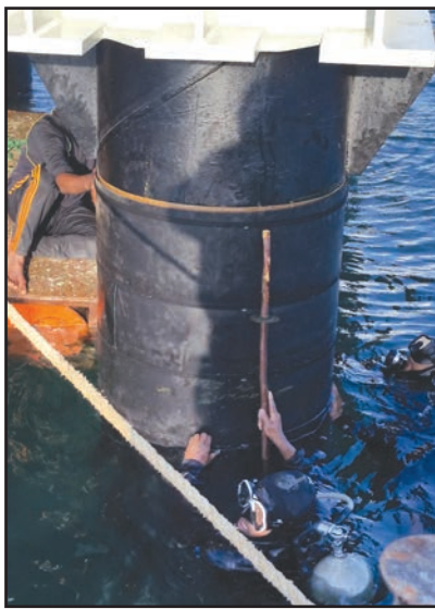
Above: The HDPE jacket is closed before being fully sealed with the banding system.
