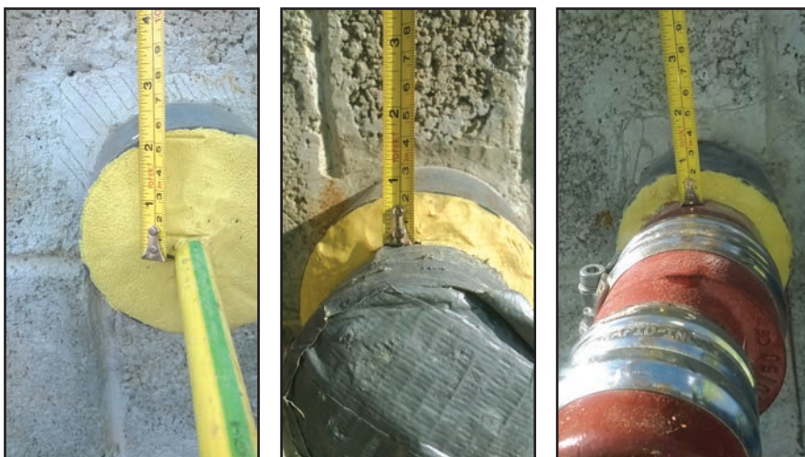
Above: To test Denso 16A thoroughly, thicknesses of between 15 and 45mm were used to seal the various pipes and cables.
