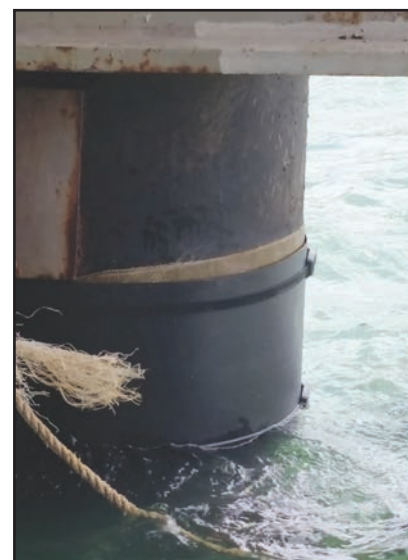
Above: The HDPE jacket is closed before being fully sealed with the banding system.
