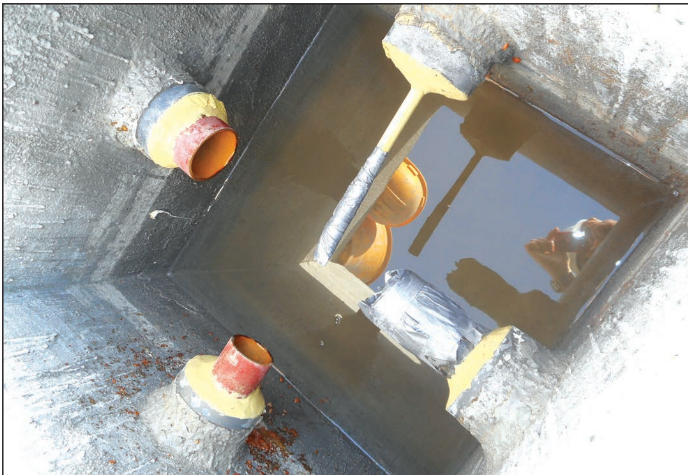
View inside the test tank showing the four entry ducts containing a mixture of pipes and cables, all sealed with Denso 16A.
