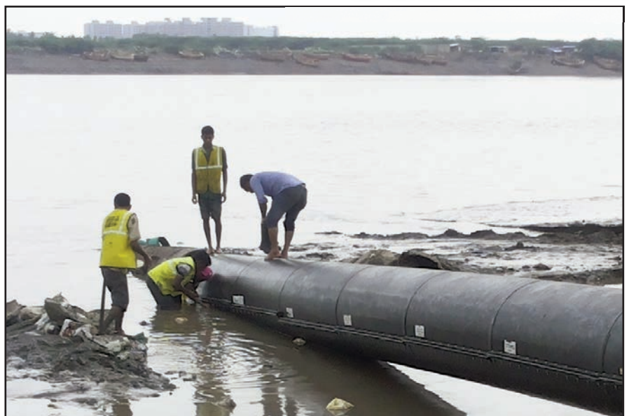
Installation of the SeaShield Series 2000 FD is almost complete.
