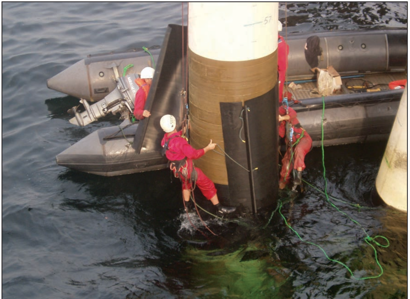
Divers fitting a 2000 FD Jacket over the Petrolatum Inner Layer on a 1.3m diameter pile.
