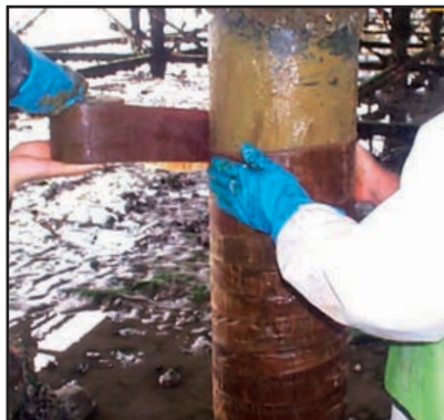
Applying SeaShield Marine Piling Tape.
