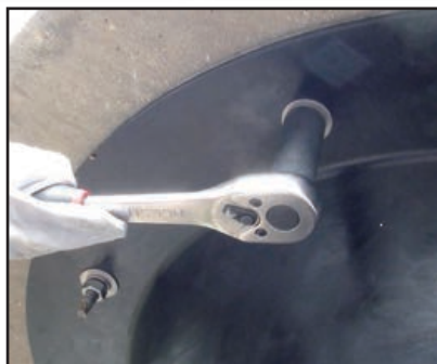
The Pile Cap is bolted to the underside of the jetty deck.
