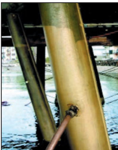
Pumping the 550 Grout. Note the visible rising level seen through the Form.
