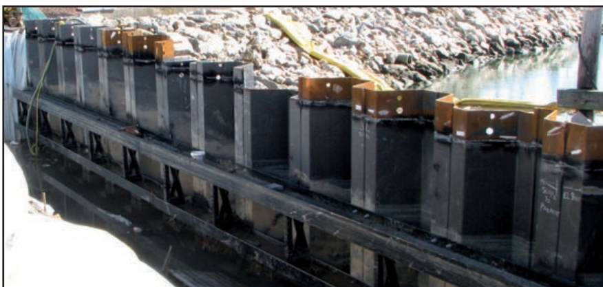
Sheet piling is coated with Rigspray prior to being driven into the ground .
