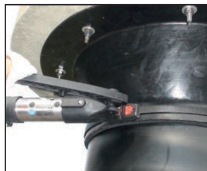
A 19mm band fixing is used to get a good seal over the existing SeaShield system.
