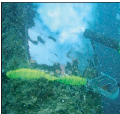
High pressure water jet under water.
