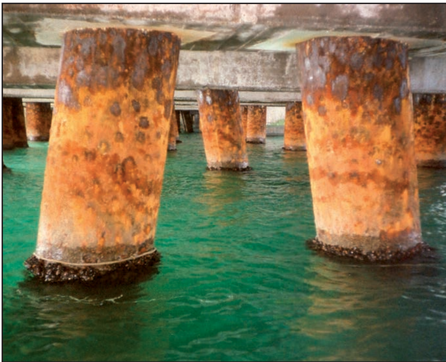
Cleaned piles ready for the application of the Petrolatum Inner Layer.
