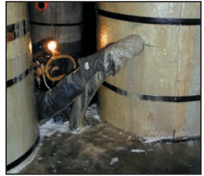
After fitting the Fiber-Forms the standard marine grout is injected by pump.
