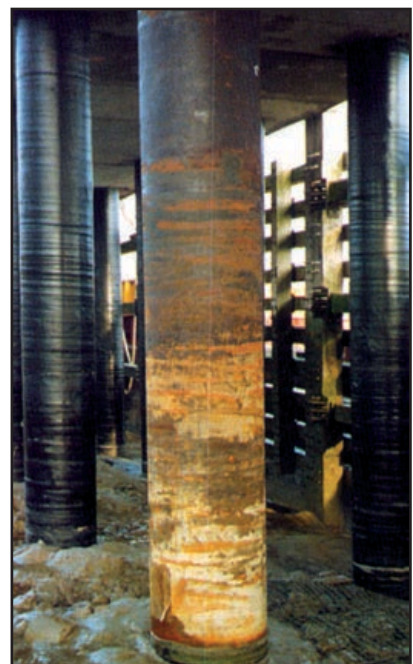
Cleaned pile ready for the application of the Seashield Series 80 System.
