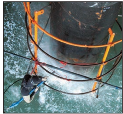
Cleaning using a high pressure water jet.
