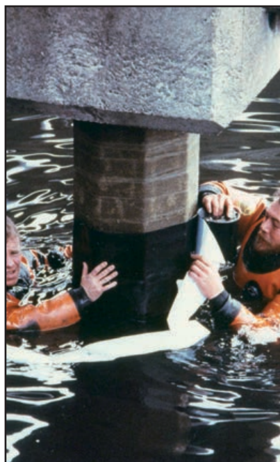
Application of Bitumen Outerwrap Tape 80 over the inner petrolatum tape layer.
