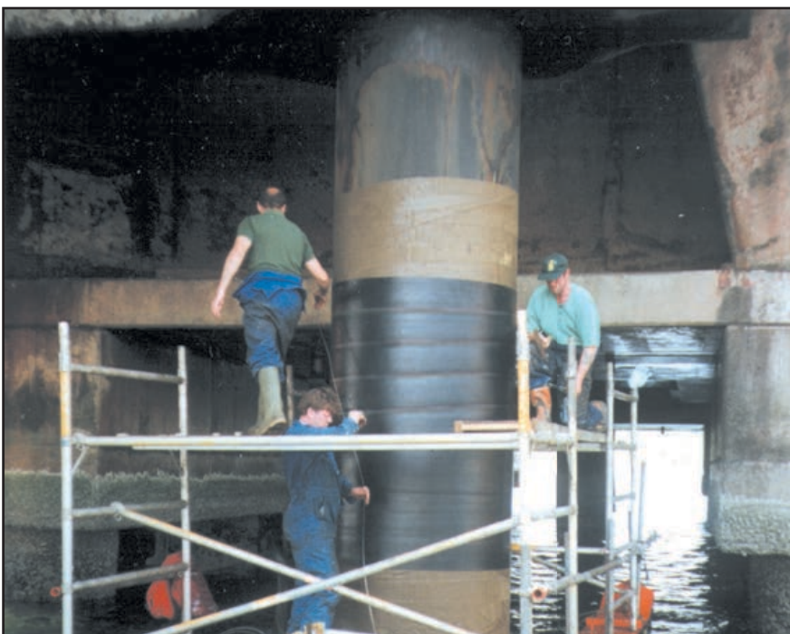
Installing the SeaShield 100 Jackets over the Petrolatum Inner Layer.
