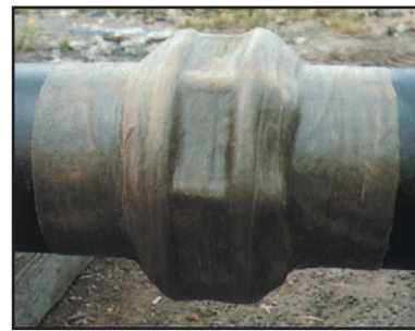
Completed coupling.
