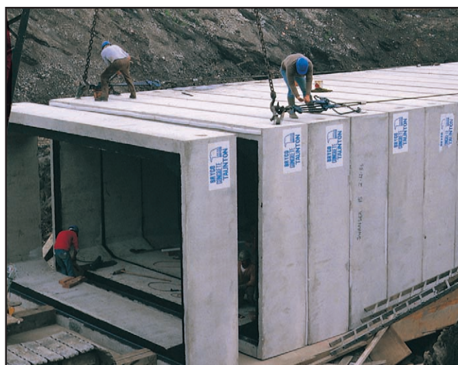
A box culvert unit is lowered into position.
