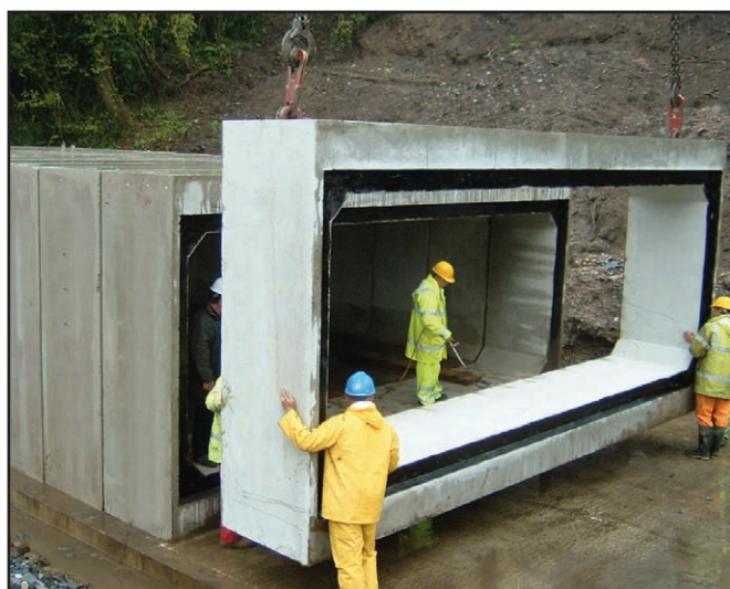
A box culvert unit is lowered into position.
