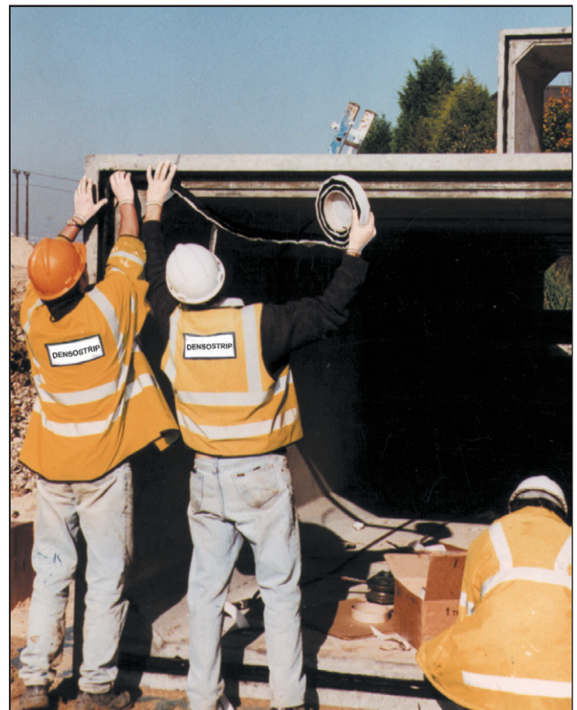
Applying Densostrip to a box culvert.
