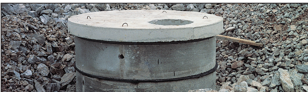
Manhole after Densostrip application.
