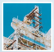
Denso Hi-Tack Tape & Primer application to all steel surface areas of a huge gantry crane. The Denso topcoat applied by brush or spray method over the Denso Hi-Tack Tape, quickly sets to form an extremely tough, uv resistant system.
