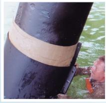
Tough outer jacket armouring installation over the applied tape in the tidal zone. Jackets pre-lined with Denso Marine Piling Tape can also be provided when rapid application is required.
