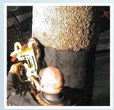
Marine growth removed by hand power tool. Petrolatum based Denso Marine Piling Tape is unaffected by high levels of chlorides and can be applied to submerged piles in fresh or sea water conditions. The tape also ensures a controlled thickness over all profiles.
