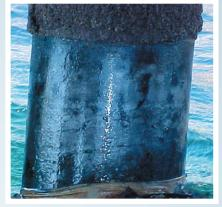
Random inspections are often carried out every 3 years (shown above). After unbolting the jacket, the Marine Piling Tape is easily removed for inspection. Refitting the tape and jacket is economical as there is no surface preparation required.
