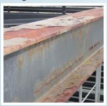
Low quality surface preparation is normally carried out by either hand power tool or High-Pressure Water-jetting methods. Denso Hi-Tack Tape & Primer accommodate thin layers of rust, moisture entrapment, smooth or rough surfaces and chemical contamination.
