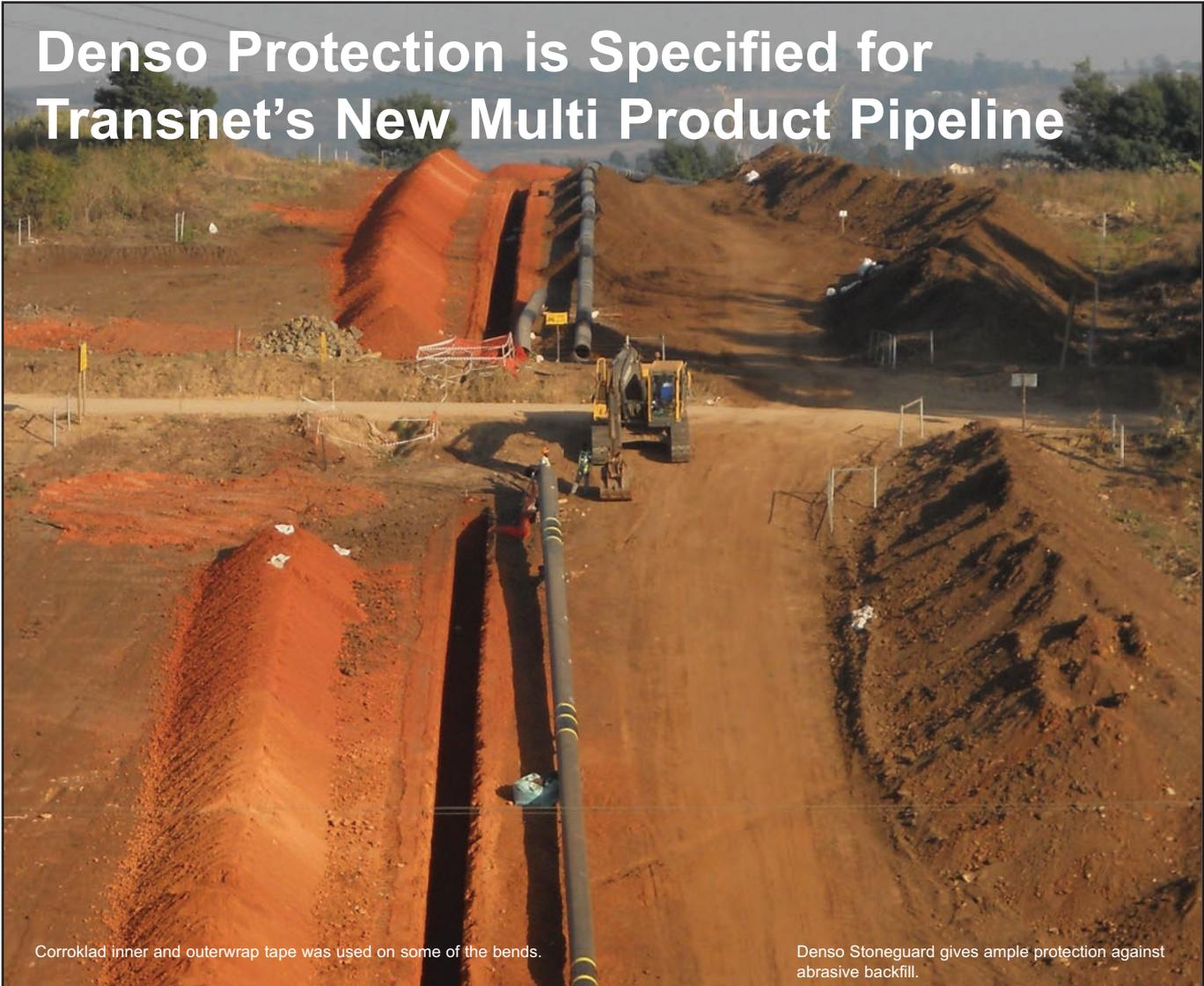
Corroklad inner and outerwrap tape was used on some of the bends.
