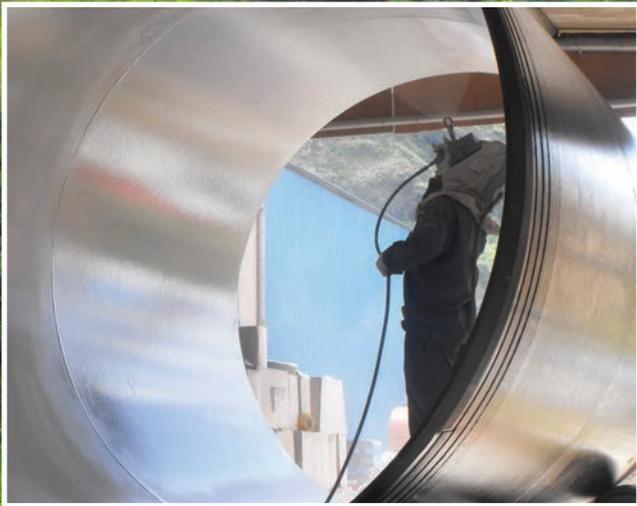
Internal surfaces of the water pipes were coated with Denso S.T. Epoxy.
