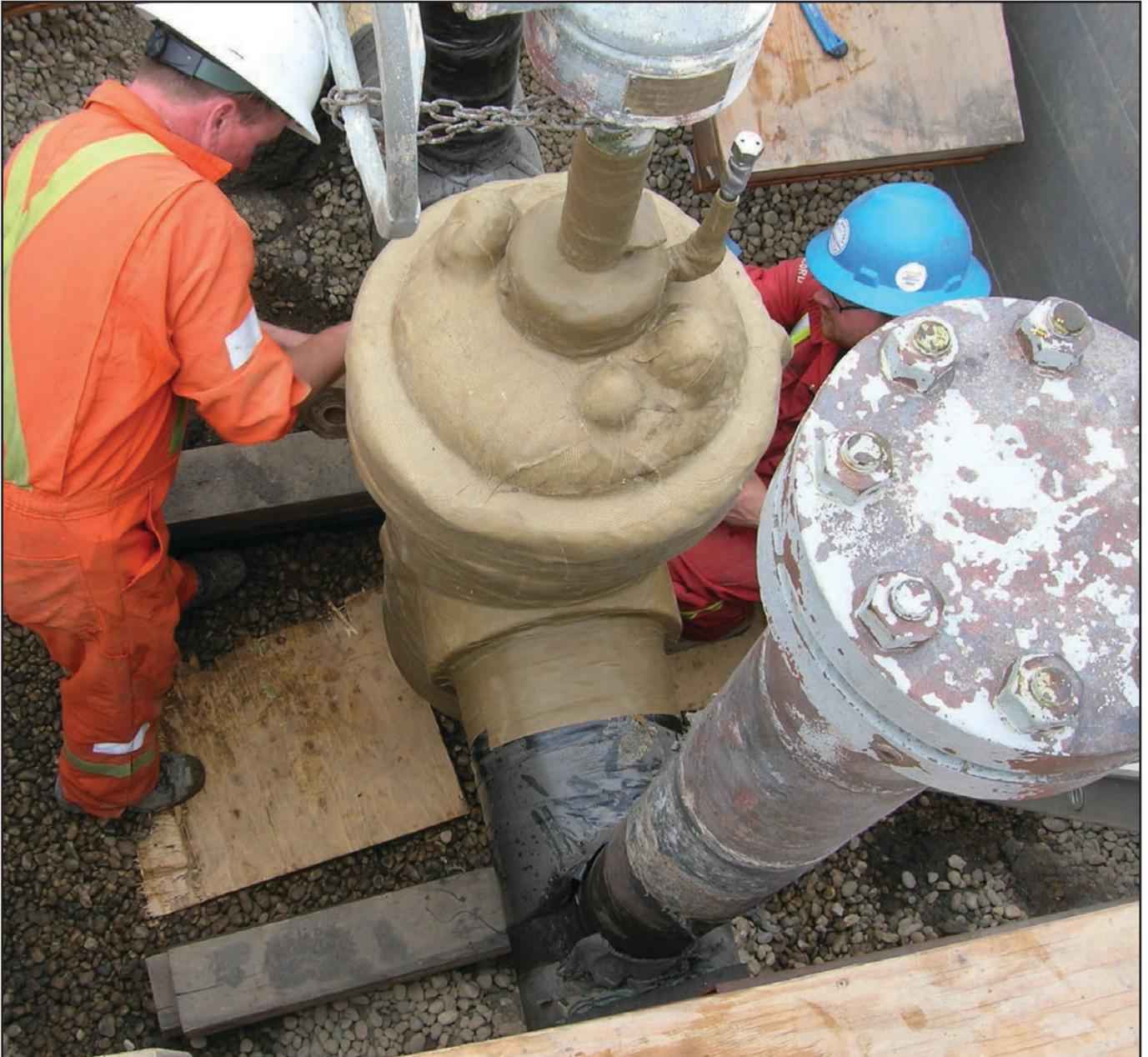
A final wrap of Denso LT Petrolatum tape to finish the job - note the flexibility of the tape and ease of wrapping over awkward shapes.
