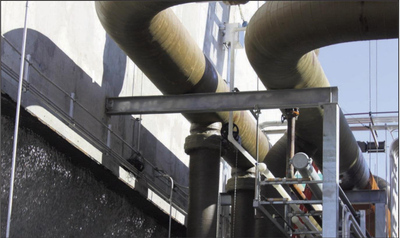
Above: Denso Paste S105 and Densyl Tape applied to all straight pipe and bends.
