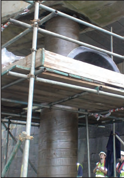
Before the Seashield 2000FD jackets and Pile Cap is fitted, the pile is wrapped with Denso Marine Piling Tape
