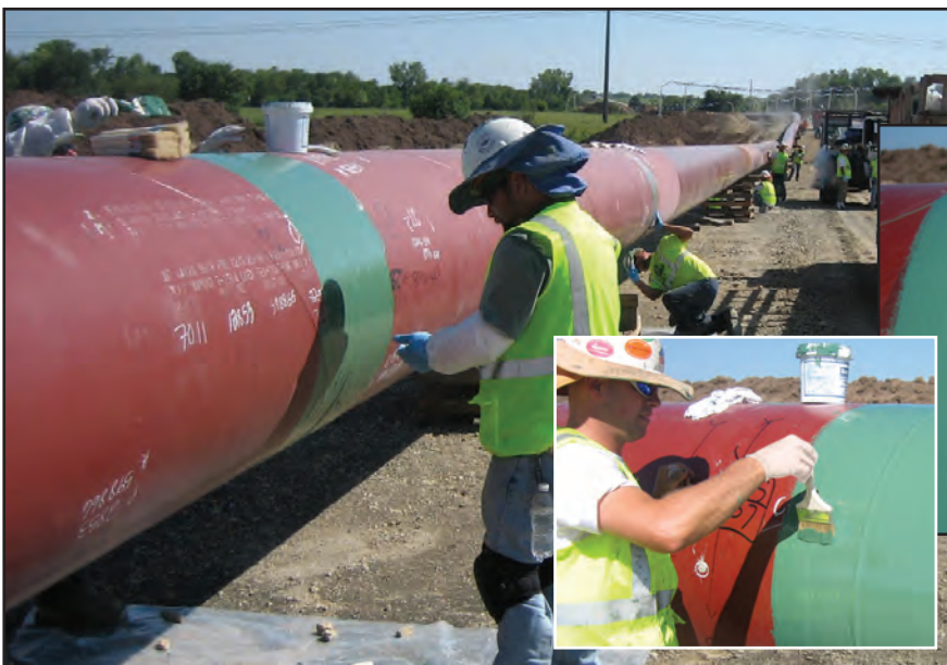
Repairing "holidays" with Protal 7200 Repair.
