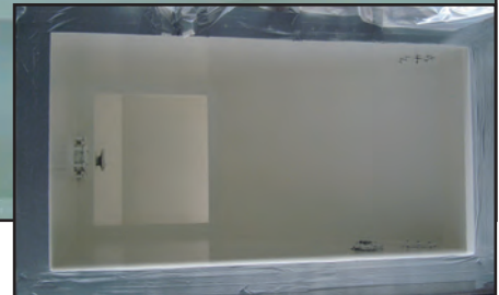
Above: All internal surfaces were coated with Denso Heatshield Special.
