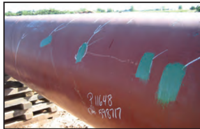
Repairing "holidays" with Protal 7200 Repair.
