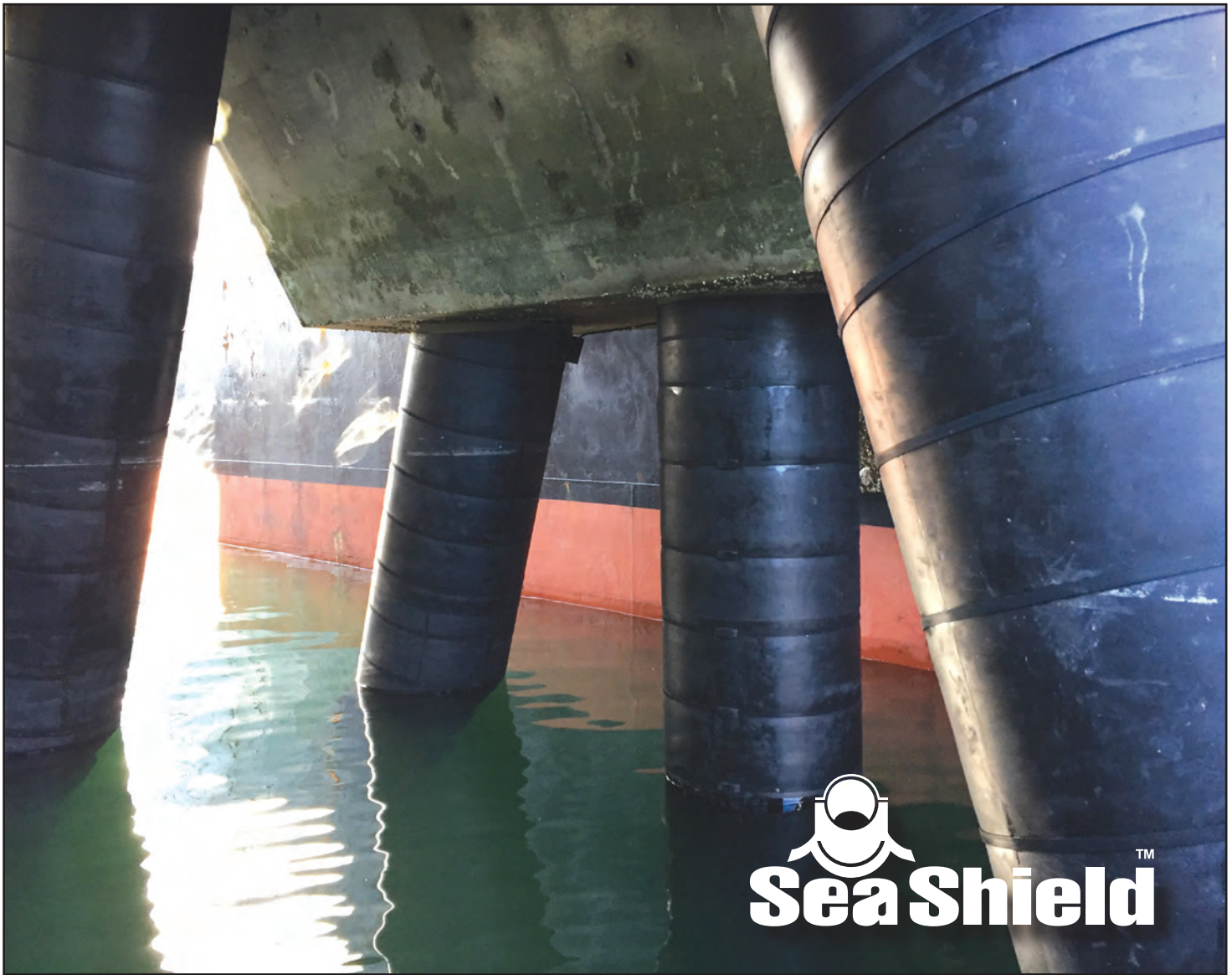
View underneath the dock showing the SeaShield Series 100™ protected piles.
