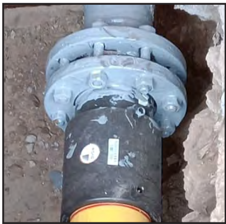
Above: A cleaned bolted flange is primed with Denso Paste™, in-situ. Below: Densyl Mastic™ is applied to fill voids and create a smooth profile on the flange before Densyl™ Tape is applied.
