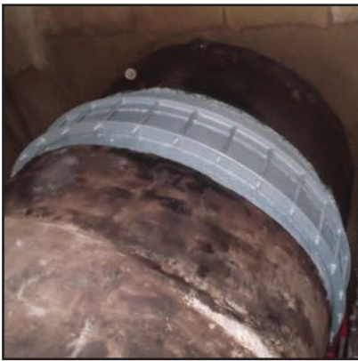
Application of paint primer.
