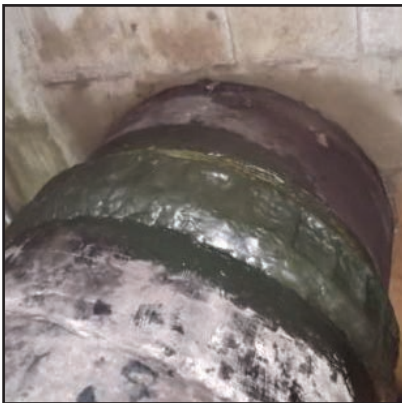
Application of Denso Mastic.
