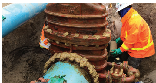
Voids and awkward angles on the valve are first filled with Denso Profiling Mastic.
