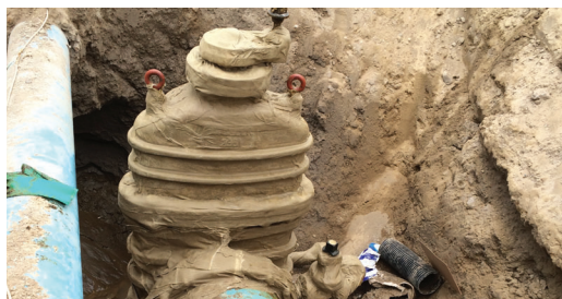
The valve is wrapped with Denso Petrolatum Tape to complete the protection.
