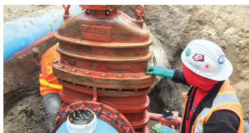
A protective coating of Denso Paste is applied by hand to provide the first layer of corrosion protection to the substrate.
