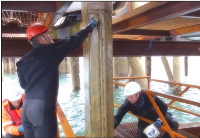
Applying the Denso Paste S105™ to a jetty pile.
