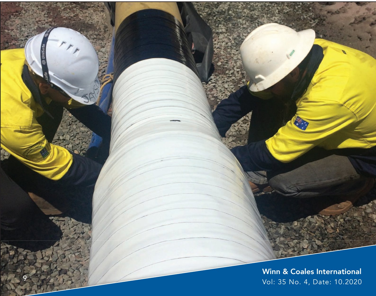
Above and below: For added protection the cured Protal 7300™ was overwrapped with the Denso S43/R23™ Self-amalgamating Butyl Tape System.
