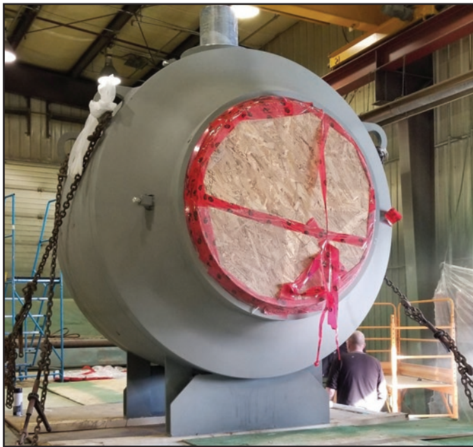
The block valves are first abrasive blasted to SSPC-SP10 / Nace 2.
