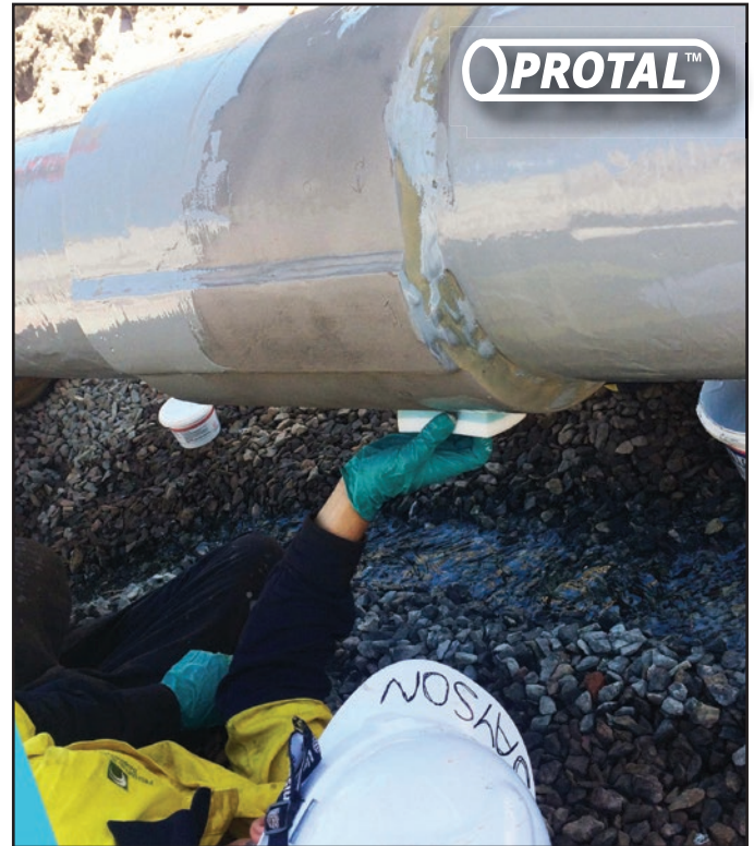
A coat of Denso Protal 7300™ was applied to a dft of 750 microns.
