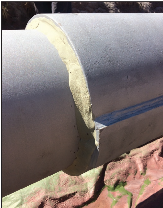
The stand-off sleeve after being welded into place was filled with a liquid epoxy.
