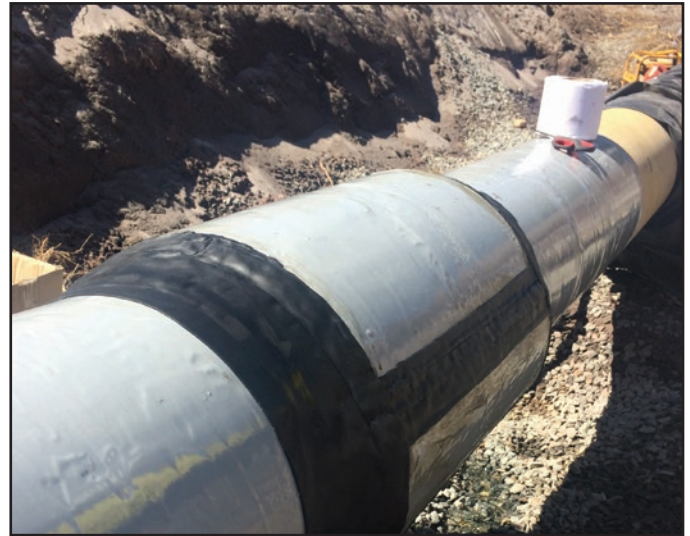
Above and below: For added protection the cured Protal 7300™ was overwrapped with the Denso S43/R23™ Self-amalgamating Butyl Tape System.
