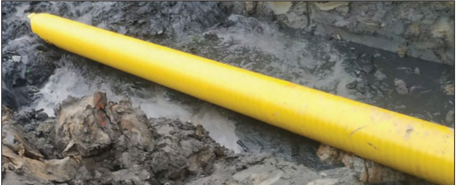
Above and below: The pipe is wrapped with Denso Marine Piling Tape™ followed by Denso PVC Self-Adhesive Tape™ for extra mechanical protection.
