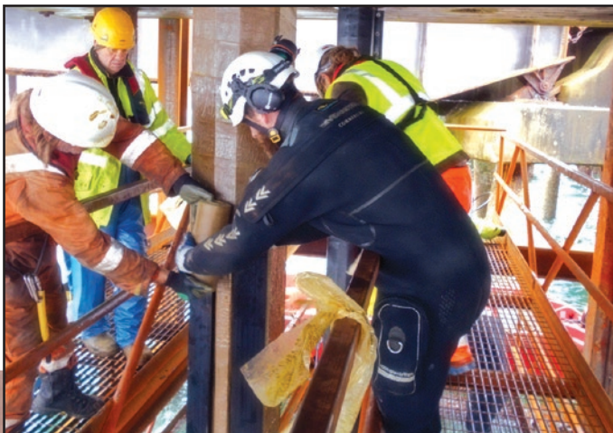
Application of the Denso Marine Piling Tape™.
