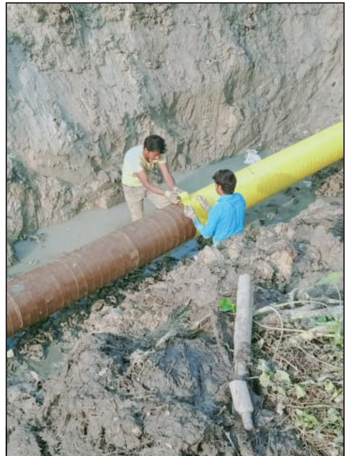
Above and below: The pipe is wrapped with Denso Marine Piling Tape™ followed by Denso PVC Self-Adhesive Tape™ for extra mechanical protection.
