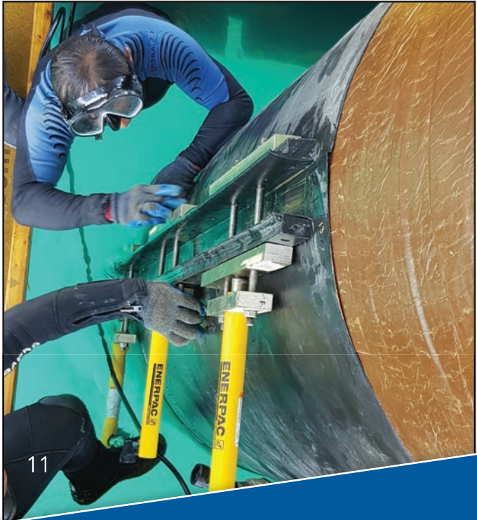
Below: The SeaShield™ Jackets are fitted and bolted together.
