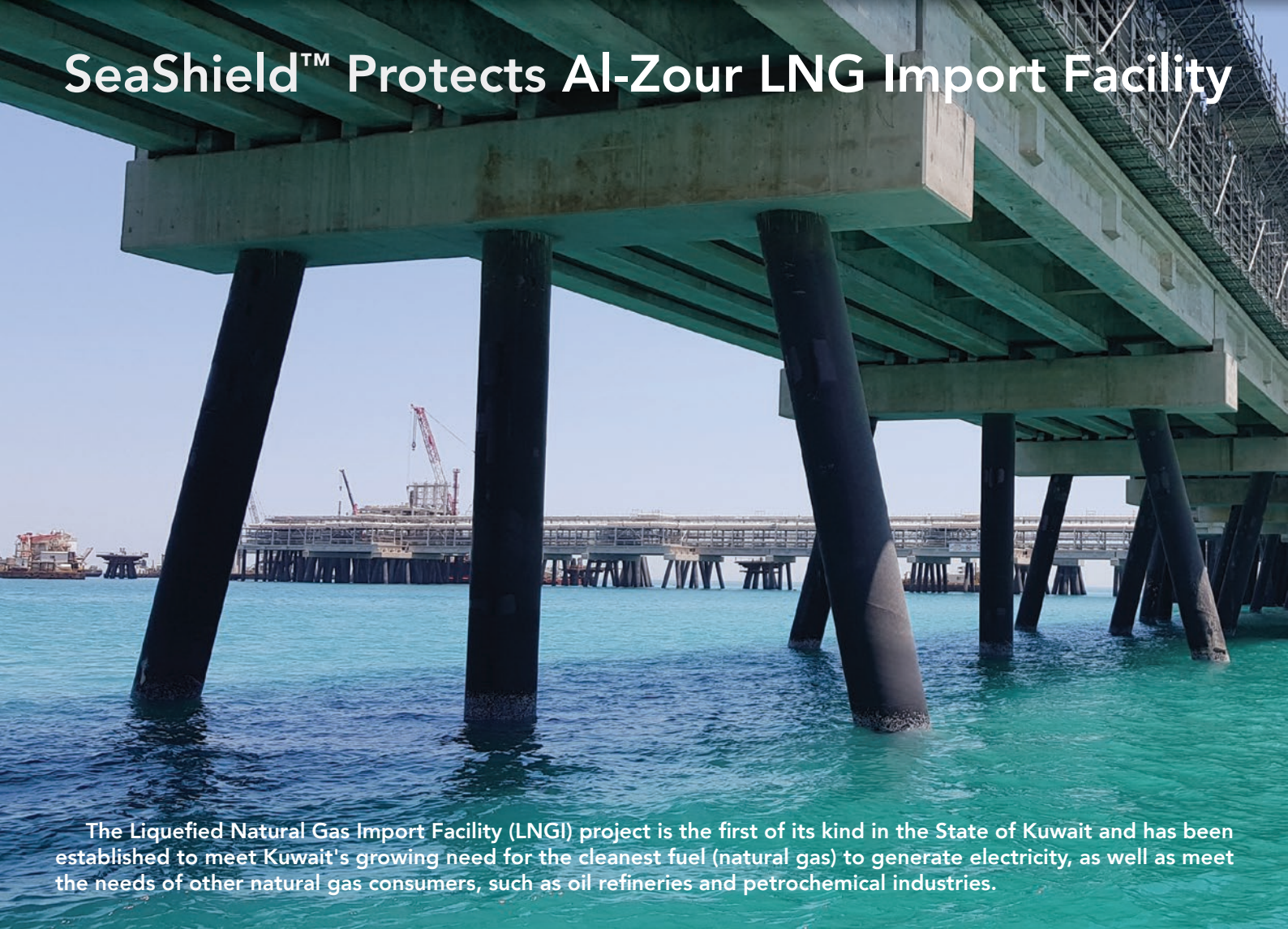
Below: The application of Denso Marine Piling Tape.
