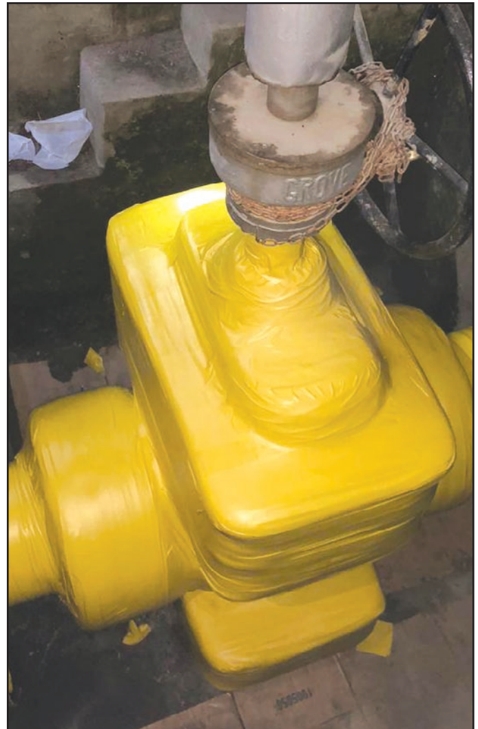
Top and bottom left: The awkward angles and crevices of a block valve are filled and smoothed prior to wrapping with Denso Profiling Mastic.
