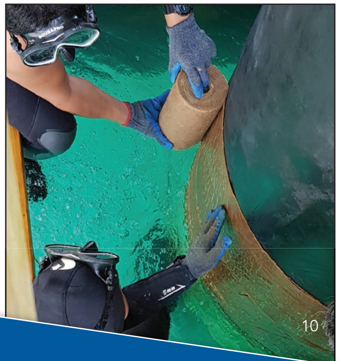
Below: The application of Denso Marine Piling Tape.
