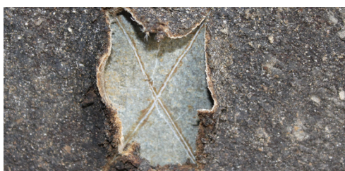
Inspection of the I-Beam, with Densyl Tape protecting since 1977, revealed the surface underneath to be in excellent condition with no corrosion.
