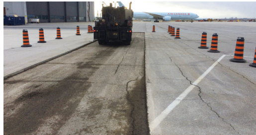
Section of taxiway being prepped for repairs.
