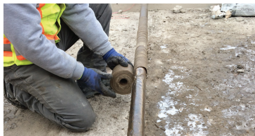
Denso Petrolatum Tape is spirally wrapped, with a 55% overlap, to complete this corrosion protection system.
