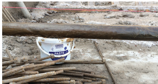
A thin layer of Denso Primer is applied to the exposed substrate prior to the application of Denso Petrolatum Tape.
