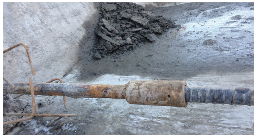
Support rod of the shoreline wall is exposed during the reconstruction phase.
